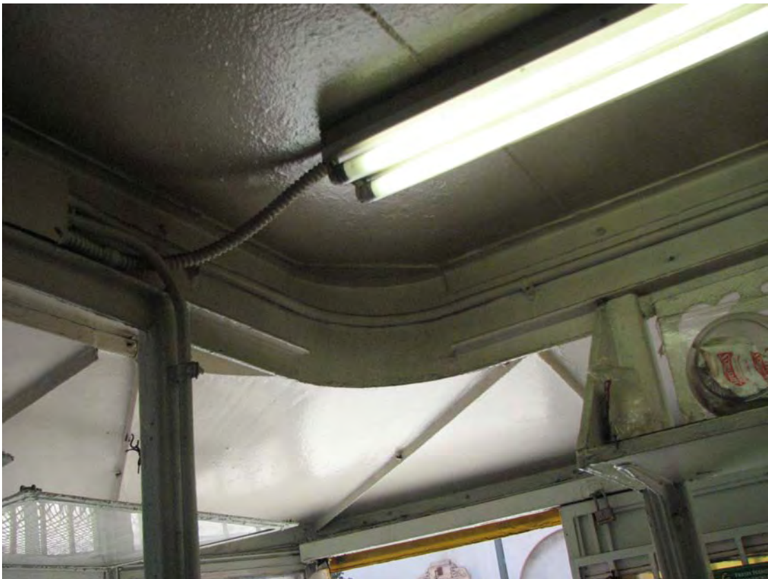
Thelma's Cafe, steel roof seen from interior, 1108 S. Broadway, July 7, 2014 (Photograph by Charles J Fisher)
