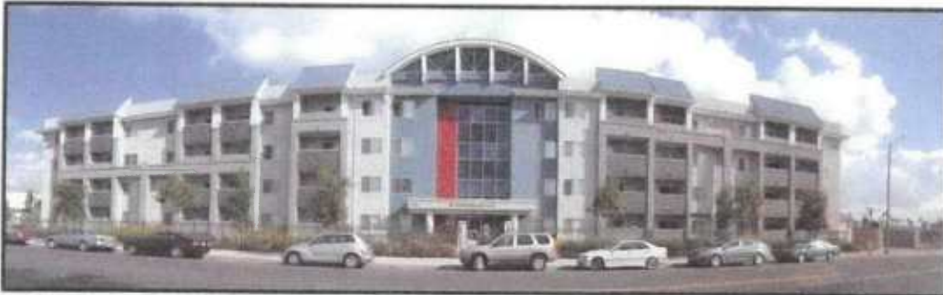
28. View of adjacent senior housing development, easterly facing from Buckingham Road.
