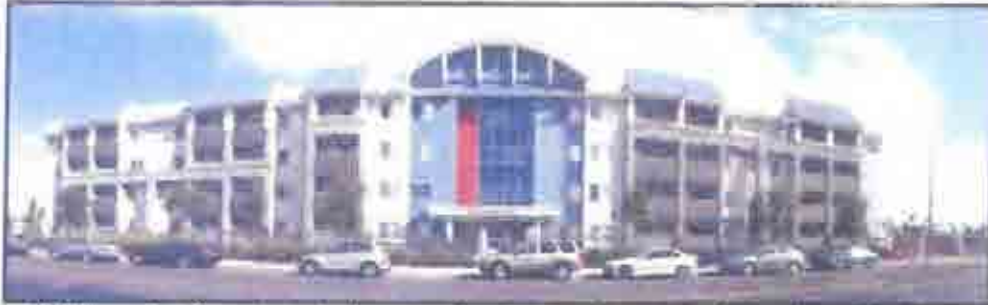
28. View of adjacent senior housing development, easterly facing from Buckingham Road.
