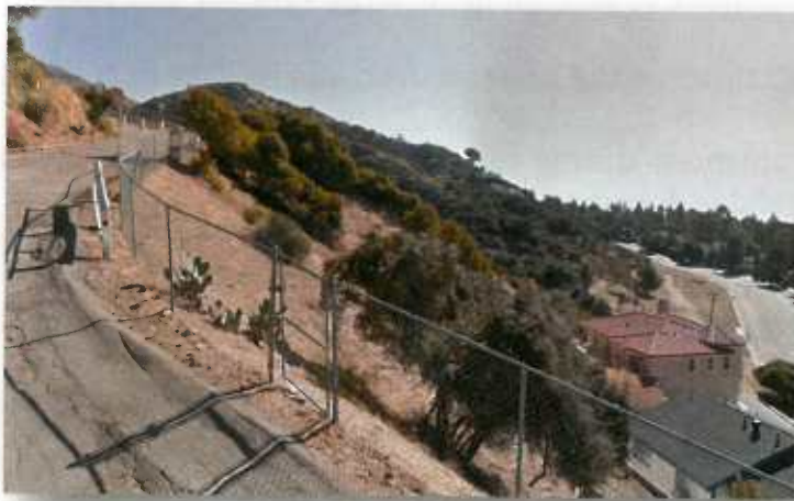
Figure 1 The building Site
