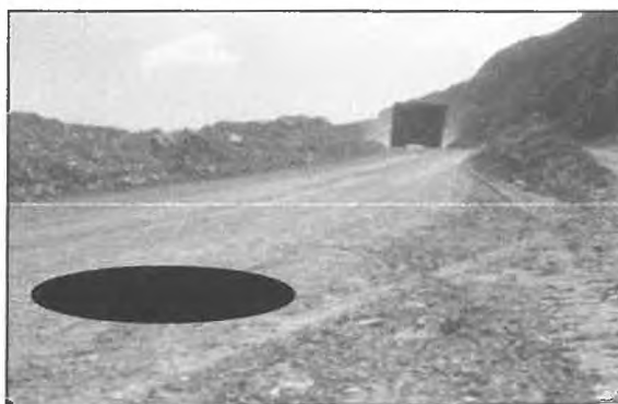
Where grades are steep, provide measures to control a runaway truck - such as berms that a truck can plow into, or escape ramps. Such features don't take the place of good maintenance, proper truck loading, and a sound driver training program, but they provide a form of safety insurance.
