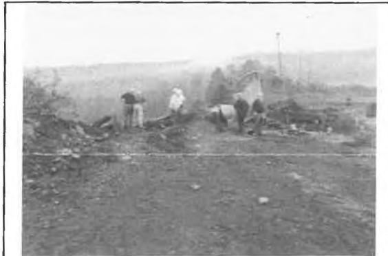
This is a close-up view of the area where the truck left the haul road...
