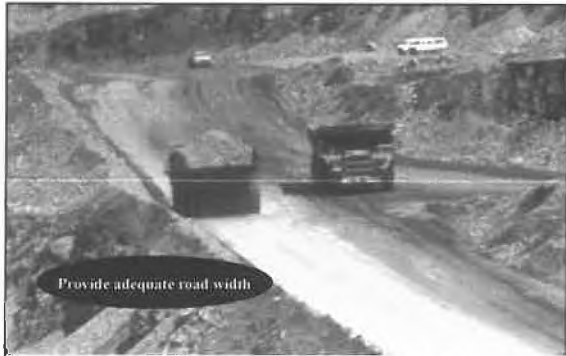
As larger trucks are used, haul roads need to be widened to provide the drivers with a reasonable margin for error. A good safety rule is to provide clearance of at least half the truck width on each side of each truck. This means that for two lanes, the haul road should be at least 3.5 times the width of the largest trucks.
