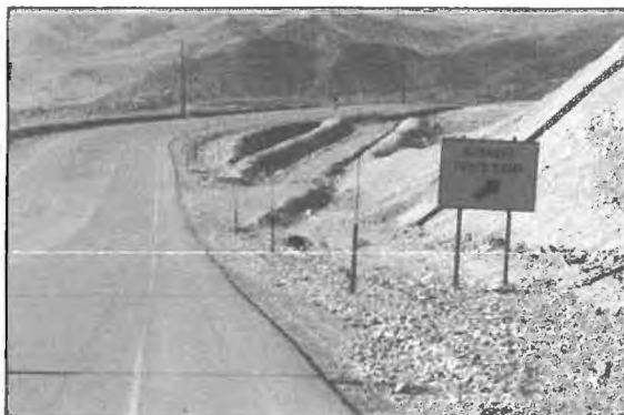
An example of a runaway escape ramp at a copper mine in Utah. A bed of loose gravel is used on the ramp to help bring a runaway truck to a controlled stop.
