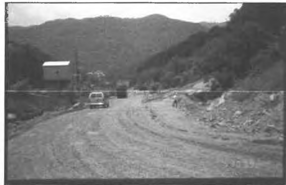
When a fatal accident occurred at this site, it was only the second time that the victim had driven down this haul road and the first time in the particular model truck. The road had an 18 % grade.
