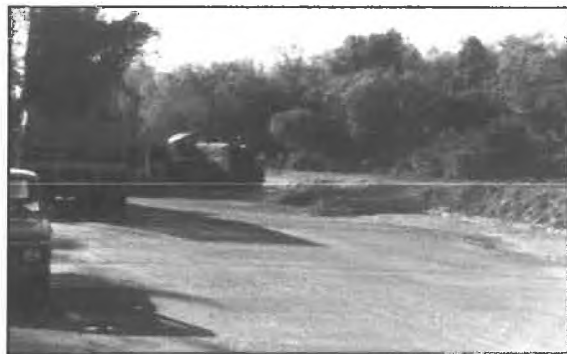
Another concern at railroad crossings - like at any type of intersection - is to ensure that the drivers have adequate sight distance down the tracks. Also avoid situations where trucks leaving mine property and waiting to enter a highway may become backed up and be sitting on the tracks. If this situation can't be avoided, train the drivers about the dangers and provide warning signs.
