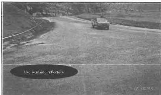
A fatal accident occurred in at this site involving a 10-ton welding truck. The welding contractor was leaving mine property around midnight. He came down this 10 percent grade to a "T" intersection. Note the skid marks coming across the intersection.
