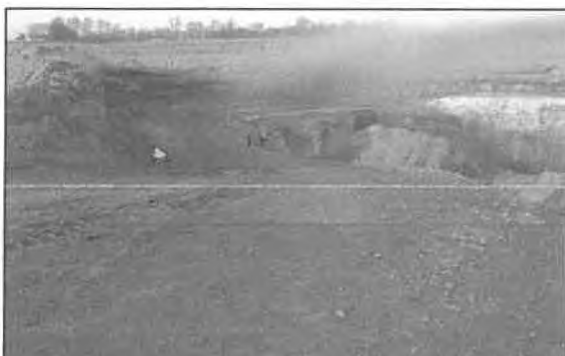
A fatal accident occurred at this mine when a scraper was hauling overburden up this ramp. The ramp was 320 feet long at a grade of 17%. The ramp runs along the top of a high wall.
