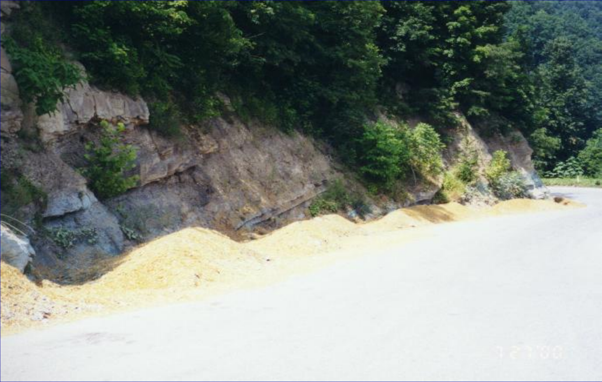
Here, loose material is placed in a “sawtooth” pattern to provide the driver with the opportunity to straddle the berm. Since the stopping power is limited, the driver must get into the berm as soon as he or she realizes there is a problem and before the truck picks up too much momentum.
