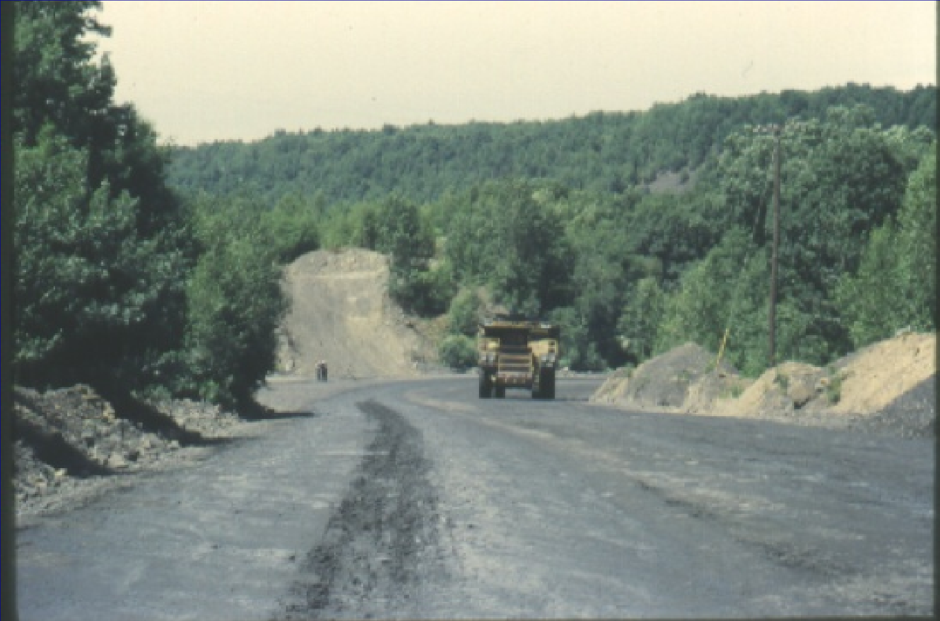
Here's an example of an escape ramp. The ramp is still under construction in this picture, but in the first year after it was completed, a runaway truck was saved on the ramp.
