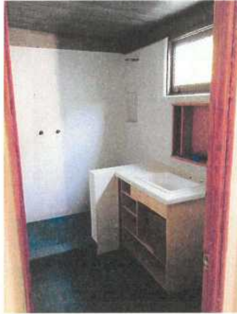
The master bathroom had been painted white and vinyl flooring installed by previous owners. Right, the in-progress restoration of the bathroom with the wood ceiling restored to the grey finish and tile floor installed, and updated the plumbing.
