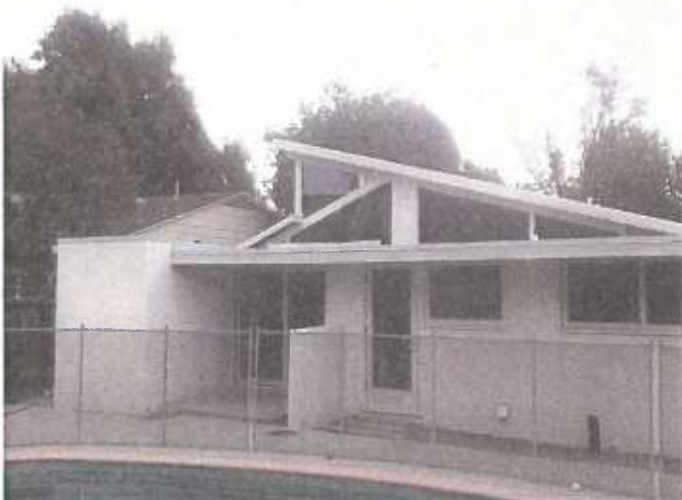
2014: the windows are no longer painted white; the large shrub has been removed to reveal the line of the shed roof; and the enclosed porch has been removed.
