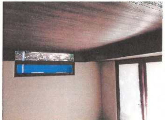
Second bedroom ceiling with restored windows and ceiling.
