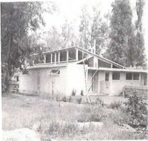
North west corner, rear exterior circa 1946-1947. The clerestory glass is transparent and awning windows can be seen on the north side of the house. Photo courtesy of the Presburger Family Archives
