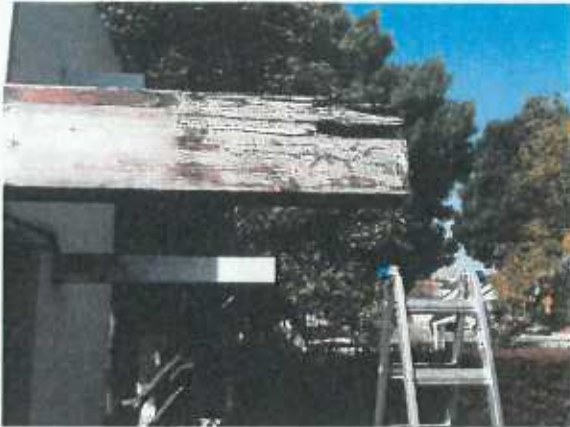
Deferred maintenance and extensive weather damage to the front overhang caused wood to weaken and rot.
