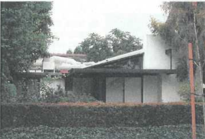
The Presburger House in 2009 at time of purchase by Culliton/Schulenberg. The sprawling HVAC system can be seen on the roof. The house was painted white with black trim, which visually "sank" the house to the ground. Some windows had been altered from the original design.
