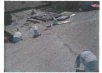
Ducting cut into the roof, seen in progress of removing the HVAC system from the roof.
