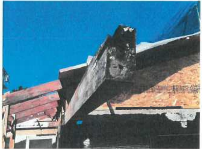
Deferred maintenance and extensive weather damage to the front overhang caused wood to weaken and rot.
