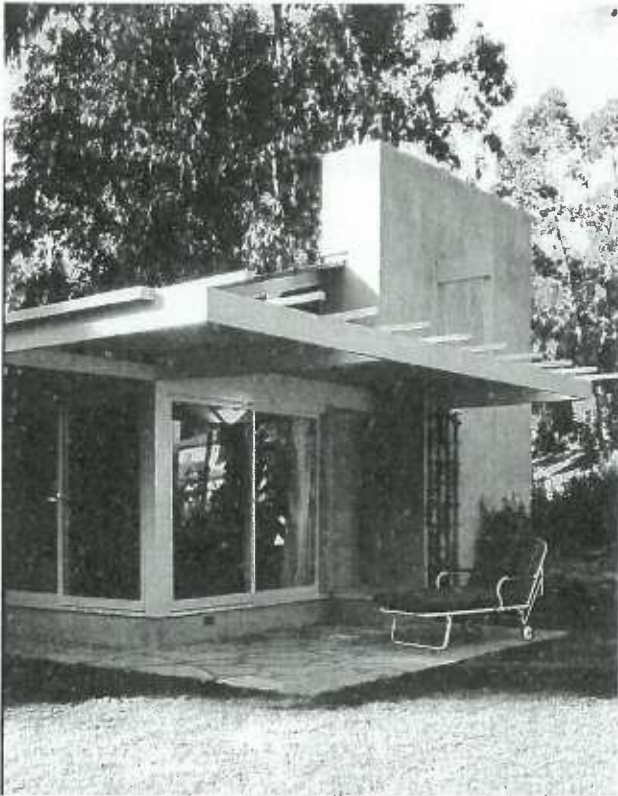
Front exterior of the living room. The overhang has been restored and the flagstone patio remains intact.
