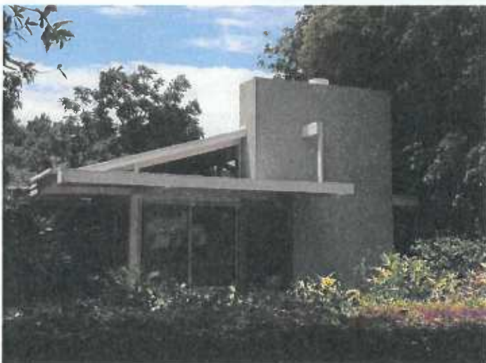
The Presburger House in 2014. Current owners restored the original color scheme which grounds the house and visually lifts the tilted shed roof. The HVAC was removed from the roof and the single plank construction Douglas Fir boards repaired. Windows and doors were repaired or reconstructed to original design.
