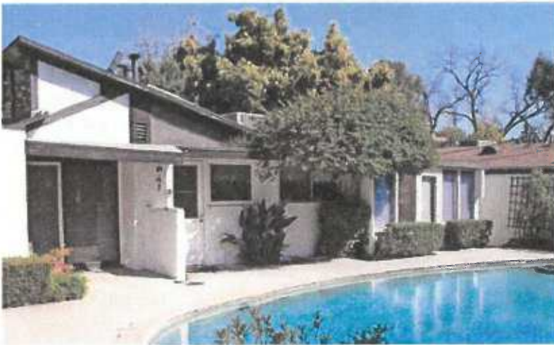
By 2009, the rear clerestory windows were painted over, the white paint and black trim blunted the visual lightness of the house, vegetation had overgrown and obscured the roofline, the HVAC was visible on the roof (top right), and the back patio had been enclosed into a dining room.
