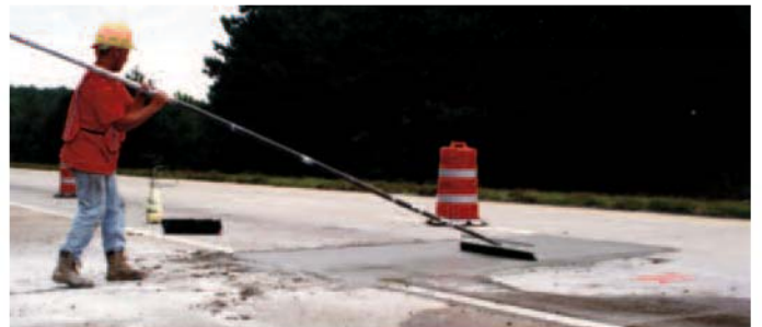
Figure 17. Texturing of a utility cut surface using a broom. Note that the curing compound is sitting nearby so that it can be applied as soon as possible.
