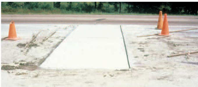
Figure 18. Proper application of white-pigmented membrane-forming curing compound. Note that the surface of the repair area is as white as a sheet of paper.
