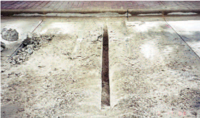
Figure 5. A pressure relief cut made using a carbide toothed wheel saw (kerf saw) down the middle of a utility cut to aid in removal of the section.
