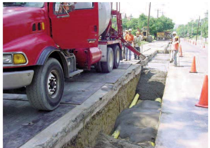
Figure 10. Placement of flowable backfill in a utility cut. Note that the flowable material is self-leveling, with the top of the backfill being placed to the base of the existing adjacent concrete slab [Photo courtesy of the Cincinnati Ready-Mix Concrete Company].
