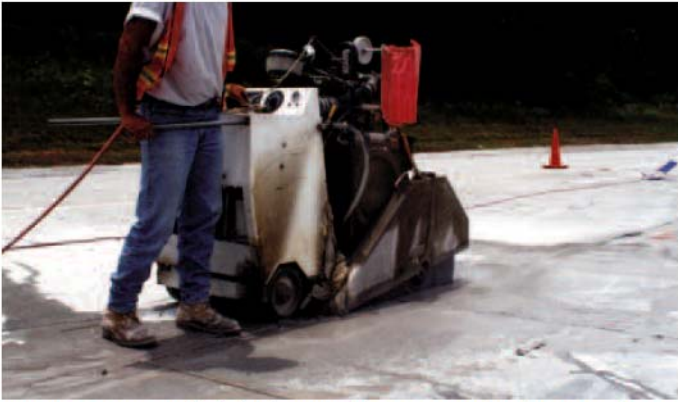
Figure 4. Diamond-bladed saw making perpendicular, straight cuts around the perimeter of a utility cut.
