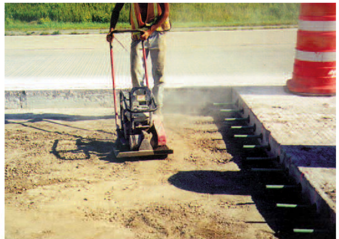
Figure 9. Recompaction of backfill immediately prior to placement of the new concrete surface course. Note that all other necessary preparation work has been completed, such as the dowel bars already having been drilled and installed.
