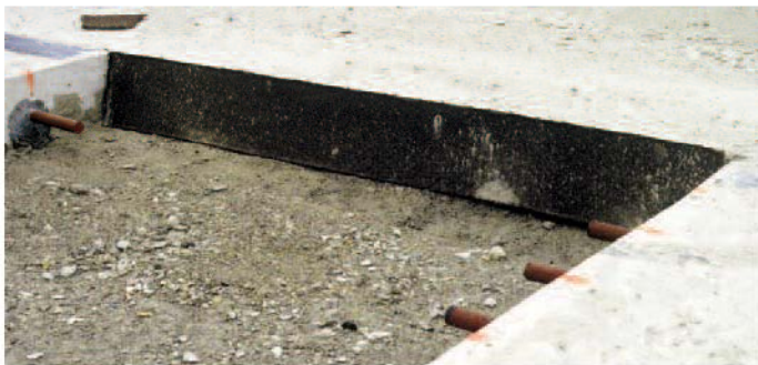
Figure 13. Fiber-board bond breaker placed along the longitudinal joint between the existing pavement and the utility cut section because the utility cut section is not longer than one slab.
