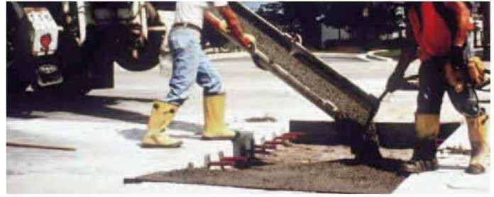
Figure 14. Proper concrete placement operations, with the concrete being discharged directly onto the subgrade/subbase inside the utility cut restoration area and a hand vibrator being used to ensure proper consolidation in the repair area and, especially, around embedded steel.
