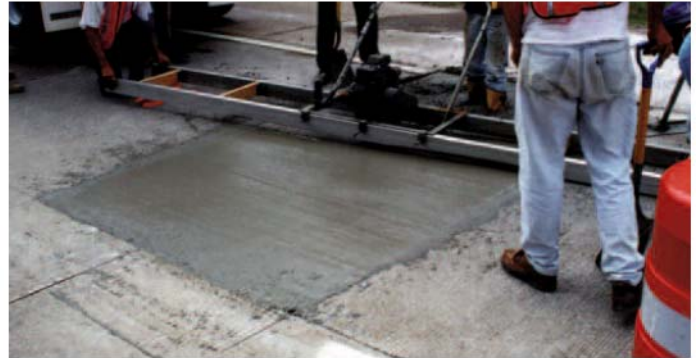
Figure 15. The new concrete surface course of a utility cut restoration being finished by a vibrating screed. Note that the surface is being finished perpendicular to the centerline because the utility cut length is less than 10 ft (3.0 m).
