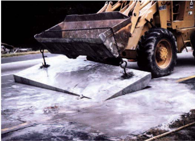
Figure 7. Partial slab removal using a lift-pin and chain lift-out method with a front end loader.
