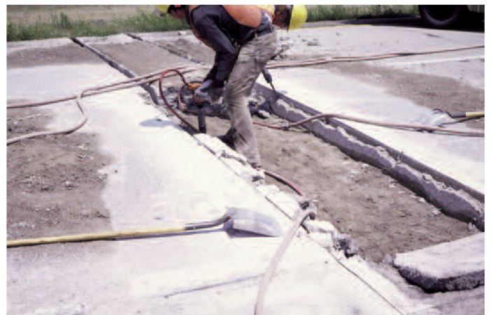
Figure 6. Breakup of a utility cut area in a concrete pavement thinner than 7 in. (175 mm) after sawing the perimeter to a depth of about one-third of the slab thickness and making two transverse full-depth kerf cuts several inches from the transverse boundaries (note the remaining slab with kerf cuts in the background) to further aid in removal of the section. Also note that the saw-cut area is being removed with light jackhammers to obtain a slightly-tapering-inward joint face on the transverse joints, without undercutting the slab.
