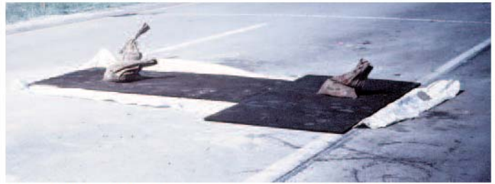
Figure 19. Insulation mats placed on top of polyethylene sheets to encourage a relatively quick strength gain.
