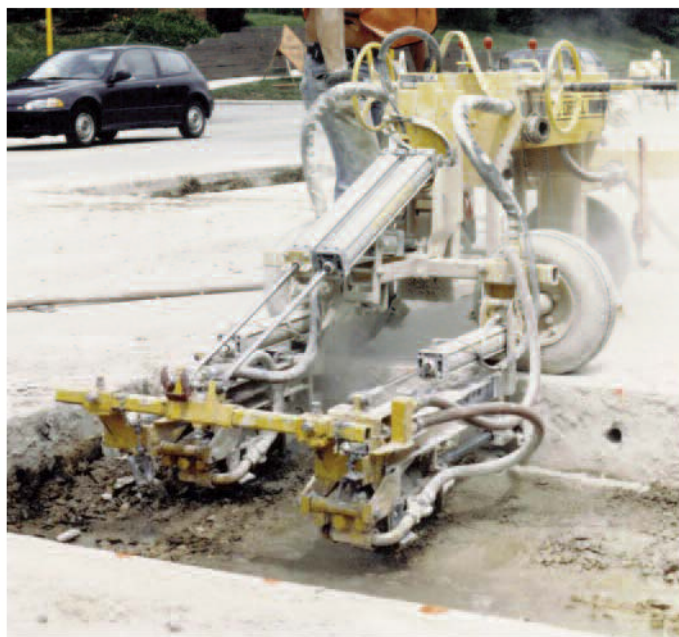
Figure 11. A gang drill, used to drill multiple dowel bar or tiebar holes simultaneously.
