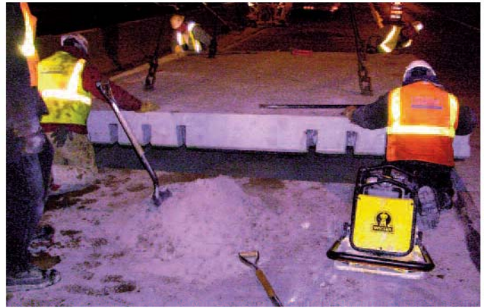
Figure 20. Positioning of a precast panel during a utility-related repair in a nighttime closure [Photo courtesy of The Fort Miller Co., Inc.].
