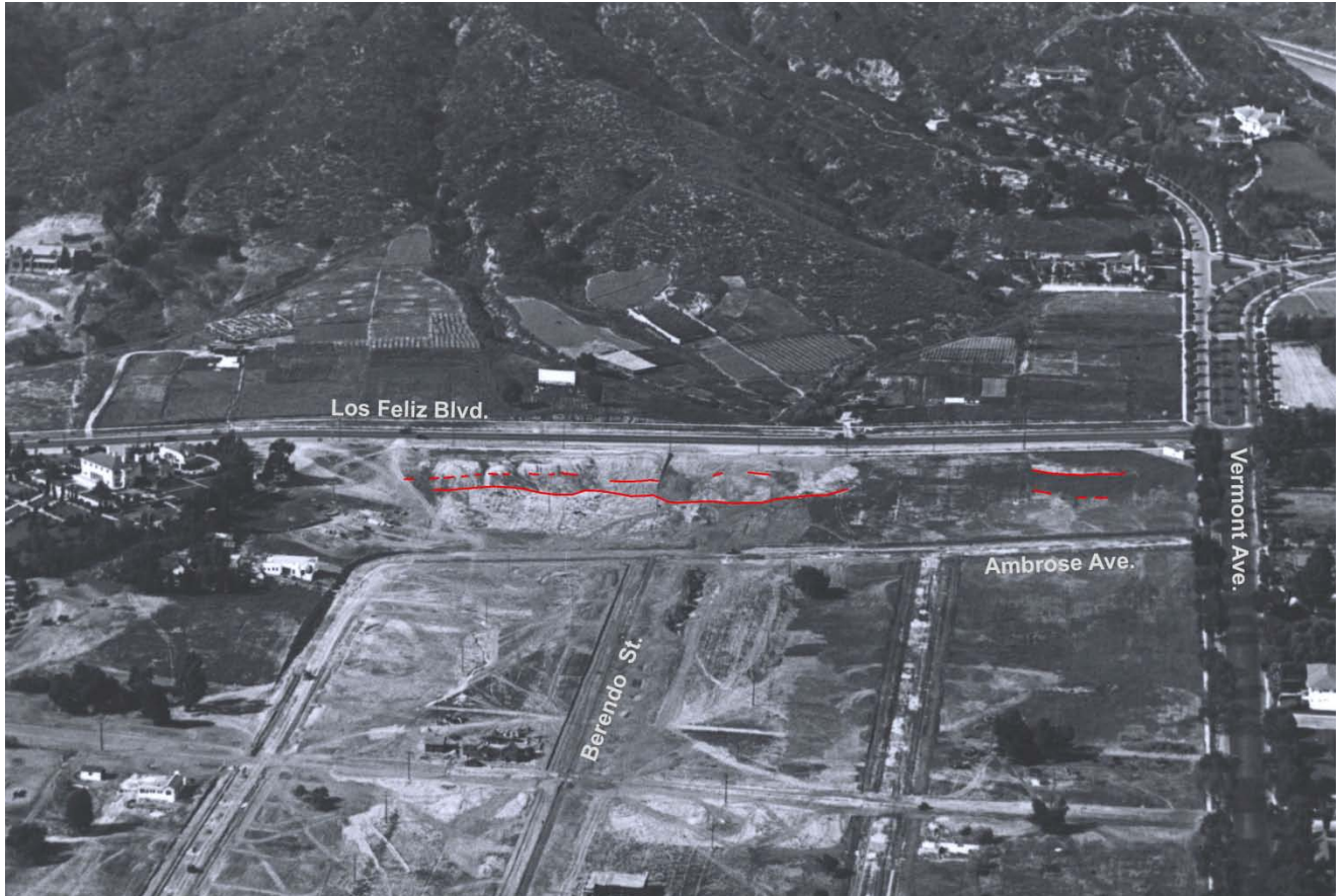
Figure 16 - Oblique aerial photo near the intersection of Vermont Ave. and Los Feliz Blvd. showing fresh grading south of Los Feliz Blvd. Lineaments (highlighted with red) are possible fault traces. (Photo by Spence Aerial Photos, circa 1921; from UCLA Spence collection).
