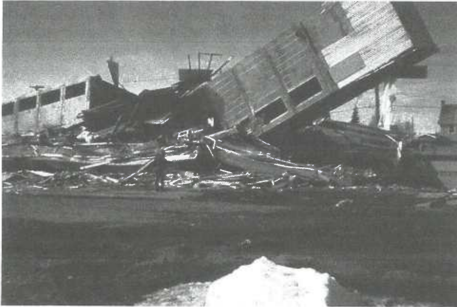
Figure 33. The remains of the Four Seasons Apartment Building, Anchorage, Alaska, 1964. The tilted column on the right was the combined elevator shaft and stairwell. (Photograph from U.S. Geological Survey Photographic Library, ID aeq00026.)
