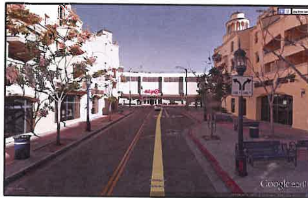
Weyburn Facade from Glendon Ave. (Mid Block)
