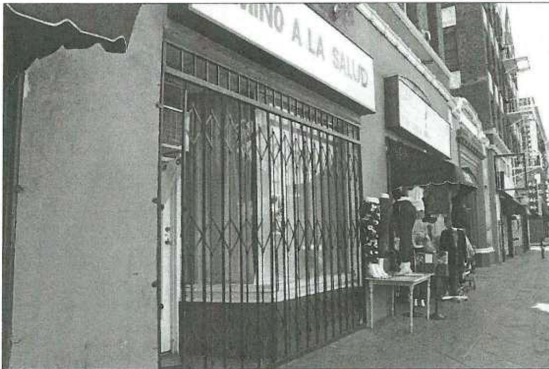
Photo 3: Haddon Hall, 3184 West 8th Street, north façade, detail of storefronts, view southwest (Chattel, Inc., 2014)
