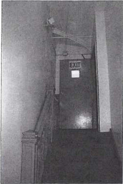
Photo 9: Haddon Hall, 3184 West 8th Street, stair from lobby, note decorative baluster and partial ceiling rib, view south (Chattel, Inc., 2014)
