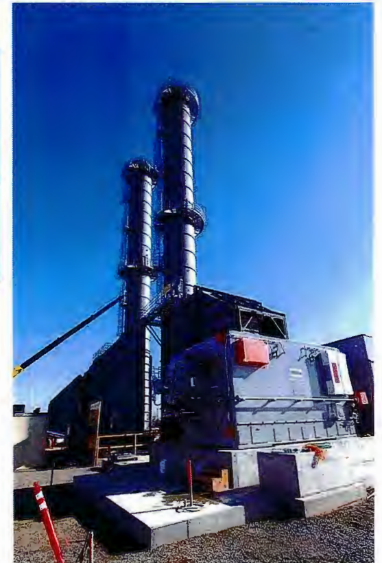
Haynes GS in Long Beach: Replaced 2 units to reduce ocean water for cooling by 50% and integrate renewables
