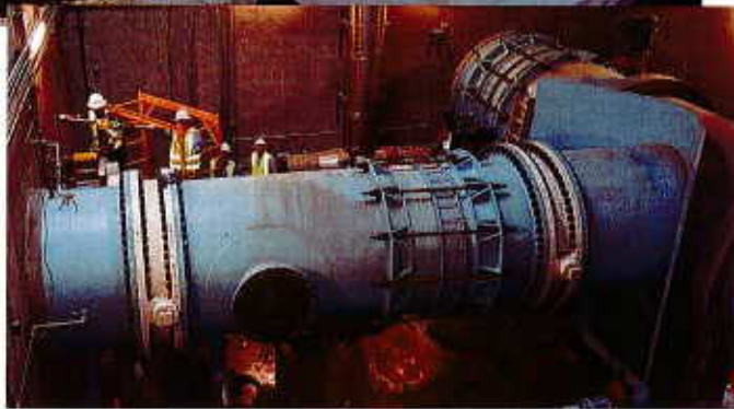
Headworks East storage facility
