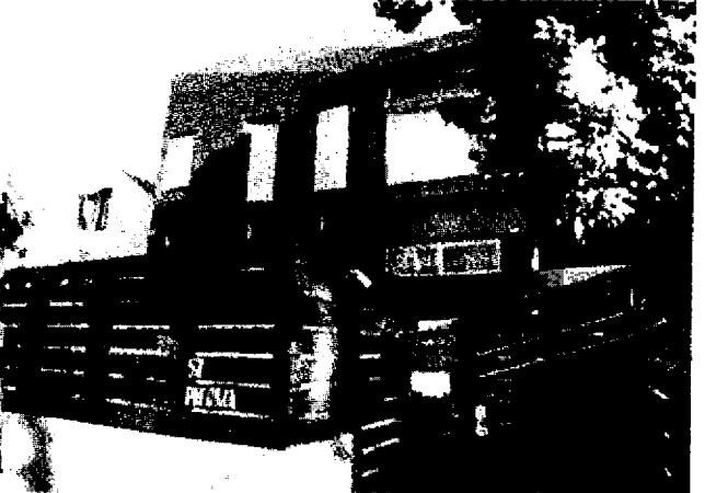
52 Paloma- 8 units RSO apartment- Mr Lambert recently purchased this building (previously Paloma 52)
