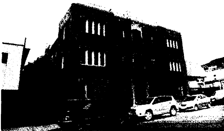
25 unit RSO apartments- Mr Lambert sold this building recently, but operates presently as Venice Ashlar Suites
