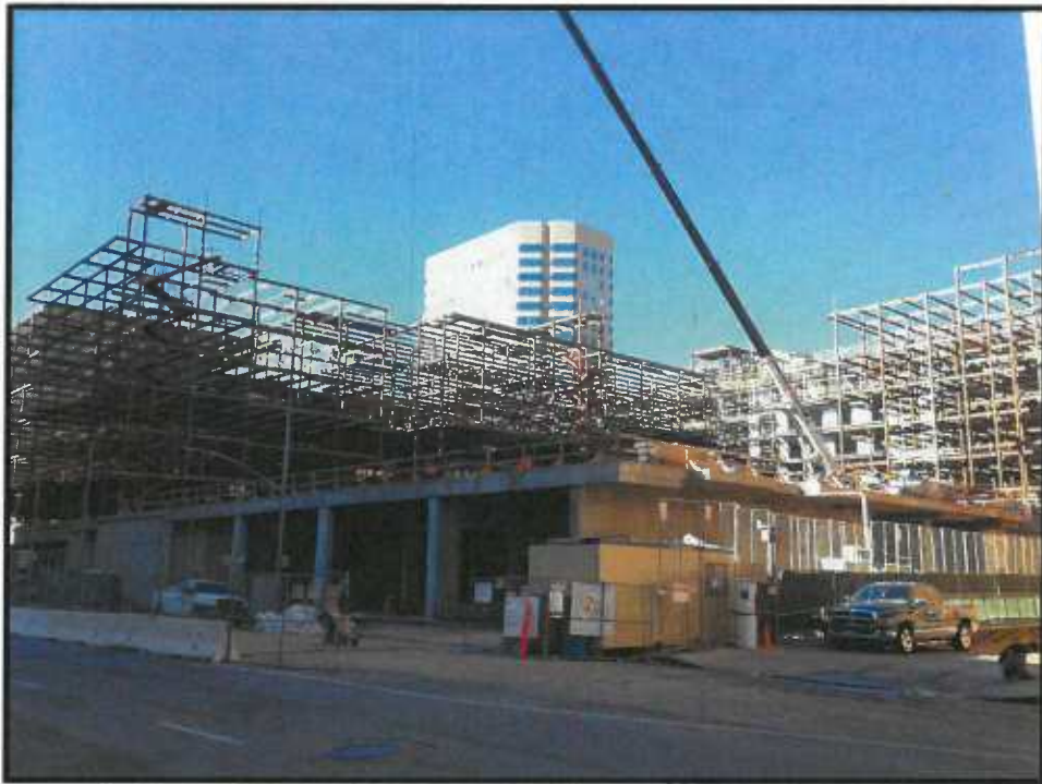
7. Project Site's Olive Street frontage, southwesterly facing
