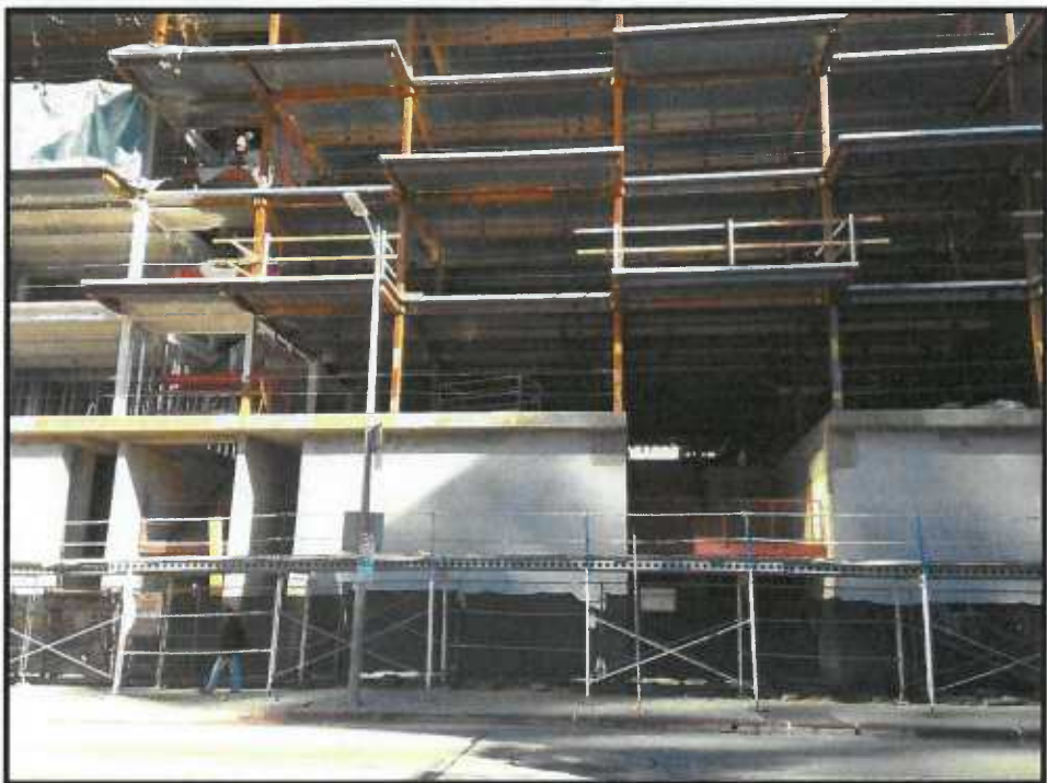
12. Project Site's Olive Street frontage (proposed Market space), northerly facing
