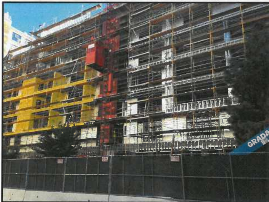
4. Project Site's Grand Avenue frontage, northeasterly facing
