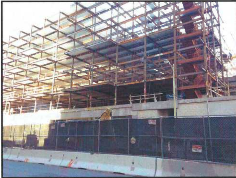
9. Project Site's Olive Street frontage, southwesterly facing
