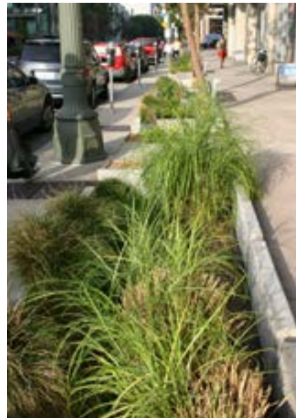
(Above and below) On Hope Street in downtown Los Angeles, several infiltration planters capture stormwater runoff through curb cuts. Stormwater enters the facility, is temporarily detained, and is treated as it slowly infiltrates natural soils.
