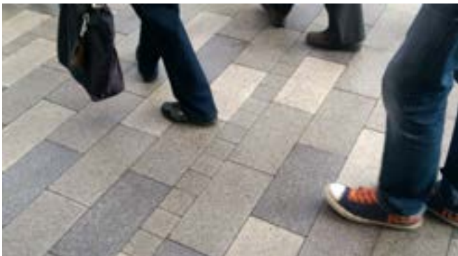
An example of permeable paving. Rainwater drains through gaps between the pavement stones.
