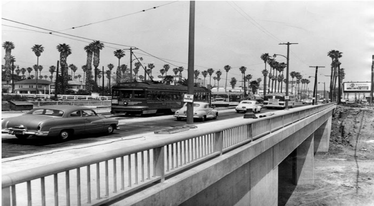
1949-1950: Hollywood Freeway under construction at Hollywood Blvd.
