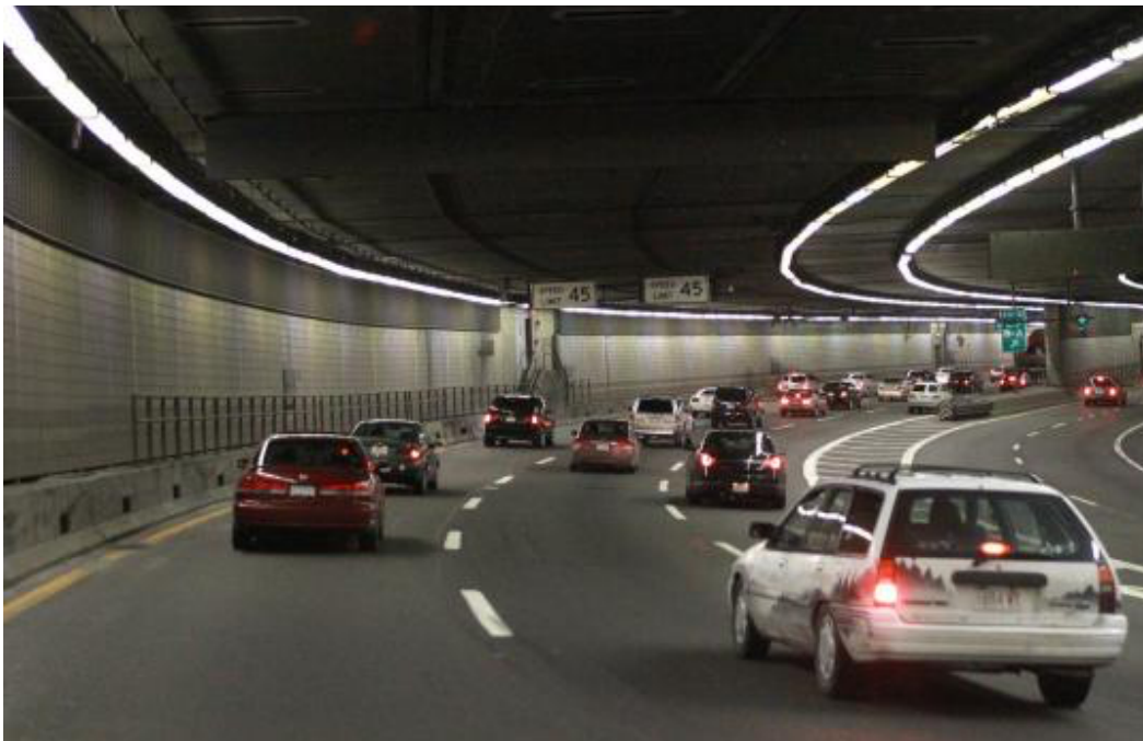
Figure 36: Ted Williams Tunnel, Boston
