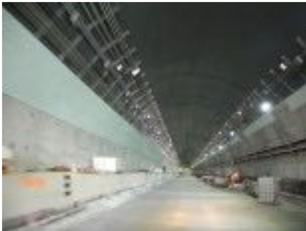
Figure 37: Port of Miami Tunnel
