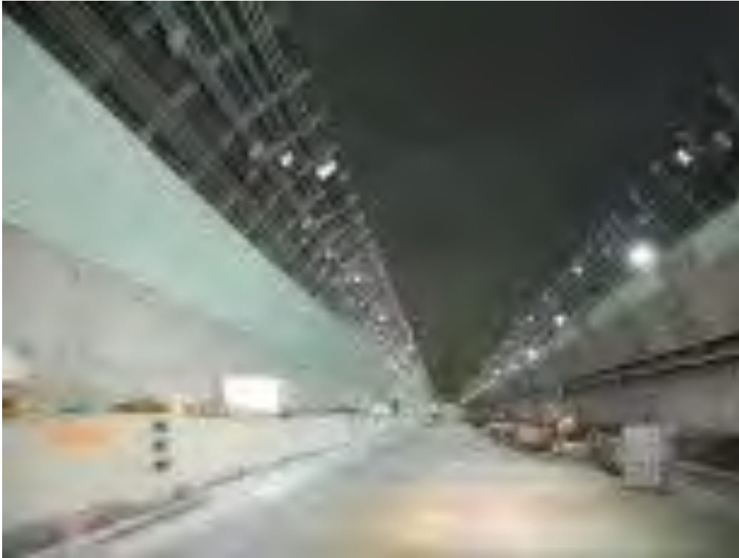
Figure 37: Port of Miami Tunnel
