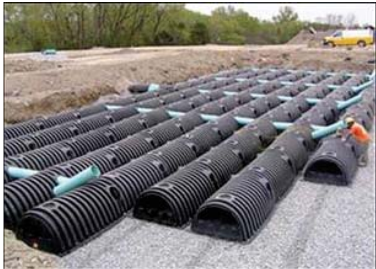
Figure 5-5: Example of StormChamber Units
