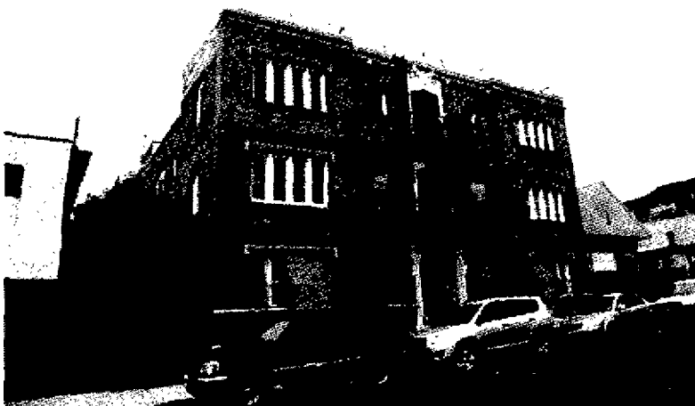
25 unit RSO apartments- Mr Lambert sold this building recently but operated previously as Venice Admiral Suites
