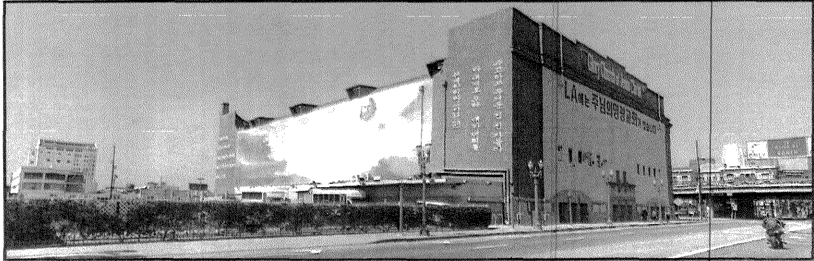
14. View of neighboring property north of subject site across Grand Avenue, northerly facing from Grand Avenue.
