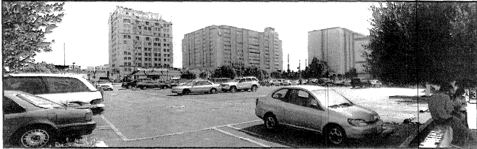
1. View of subject site, southerly facing from the northwestern corner of subject site along Grand Avenue.
