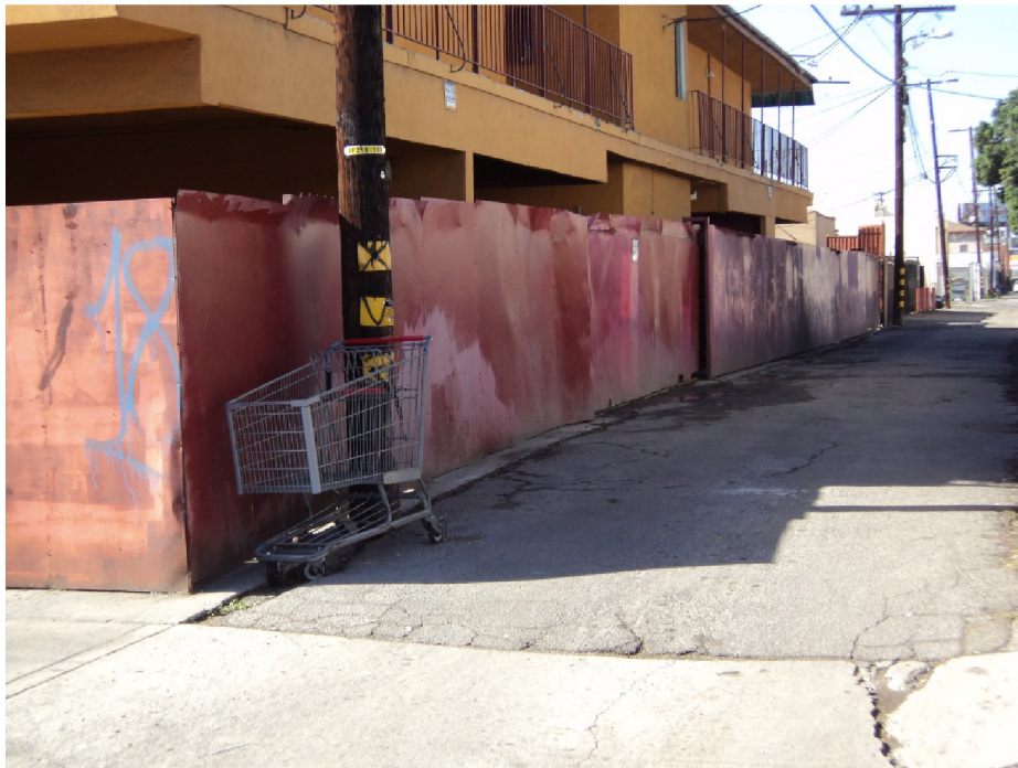
Motel from alley looking southwest
