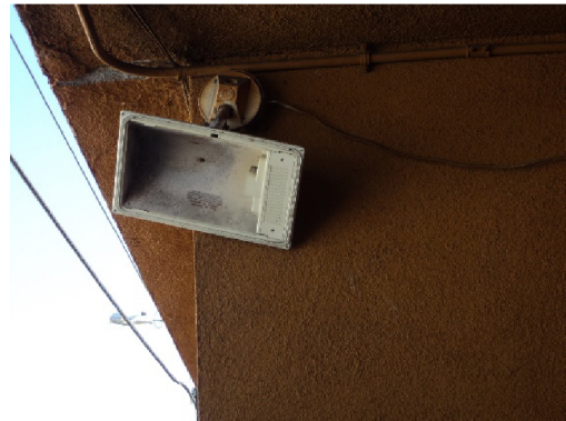
Broken light fixture
