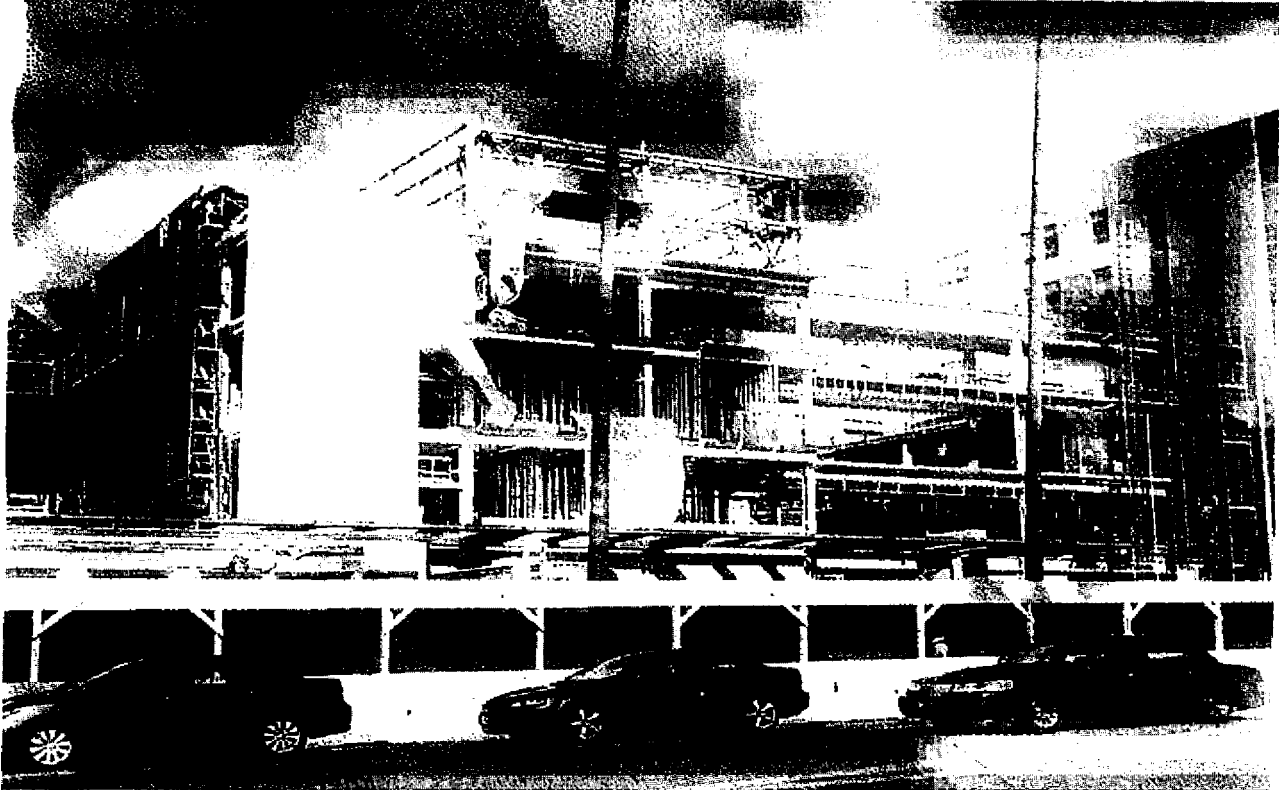
Kaiser Permanente Hospital's ongoing reconstruction, as required by State and Federal law.
