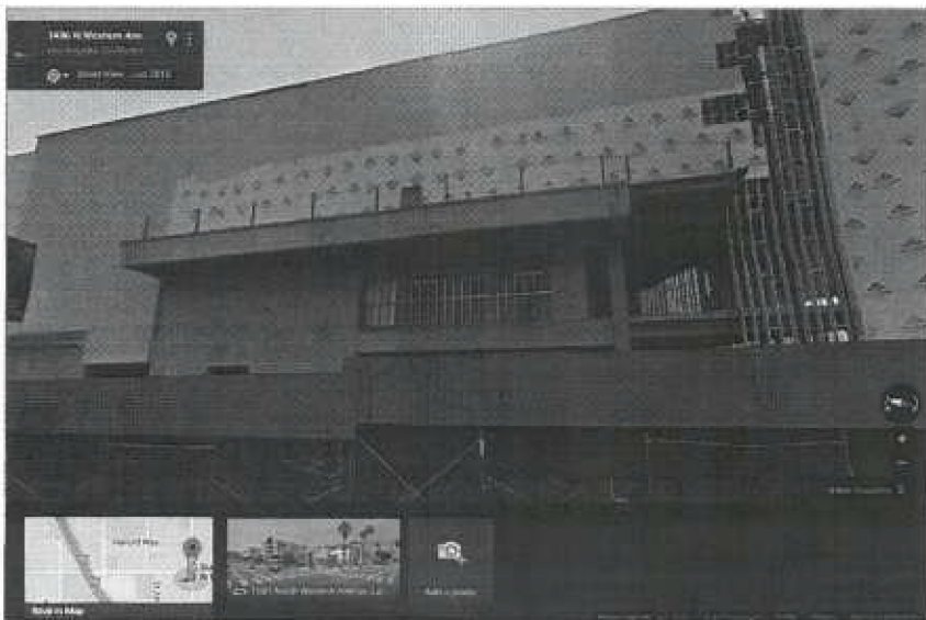
Photo showing that existing Target building is comprised mainly on the third level of fiberglass foam board and non-structural metal studs.
