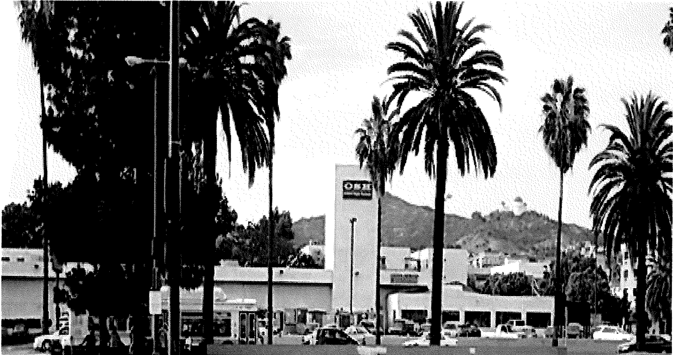
Immediately north of the Target site: A former one-story OSH Hardware store, now WSS Shoes.
