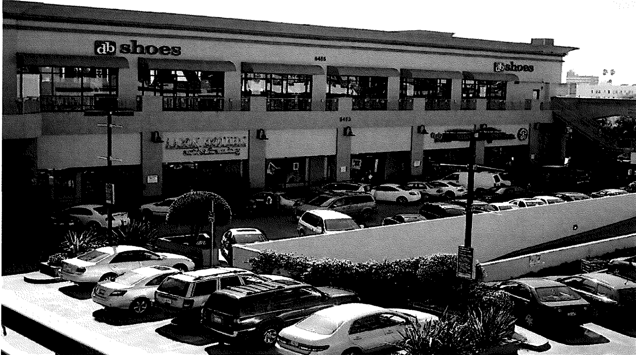
Inner plaza at mixed-use development offers various neighborhood-serving retailers.
