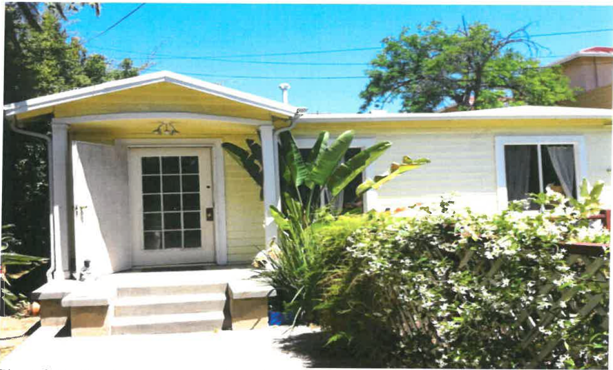
Photo above: Rear house constructed in 1920.
