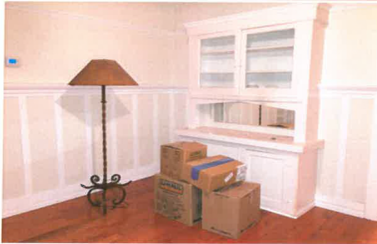
Dining room built-in floor-to-ceiling breakfront at north wall, bat and board with baseboard & plate rail; original wood floor, at 4513 Russell Avenue, photographed June 2015.
