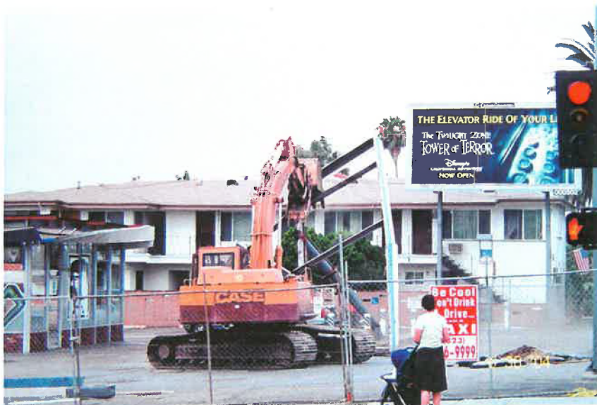
Image dated from 2004 showing the demolition of the same gas station.
