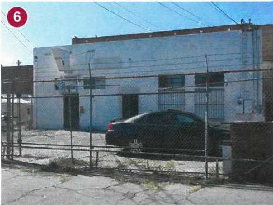
6 Parking Lot, facing rear of subject site. Direction: North
