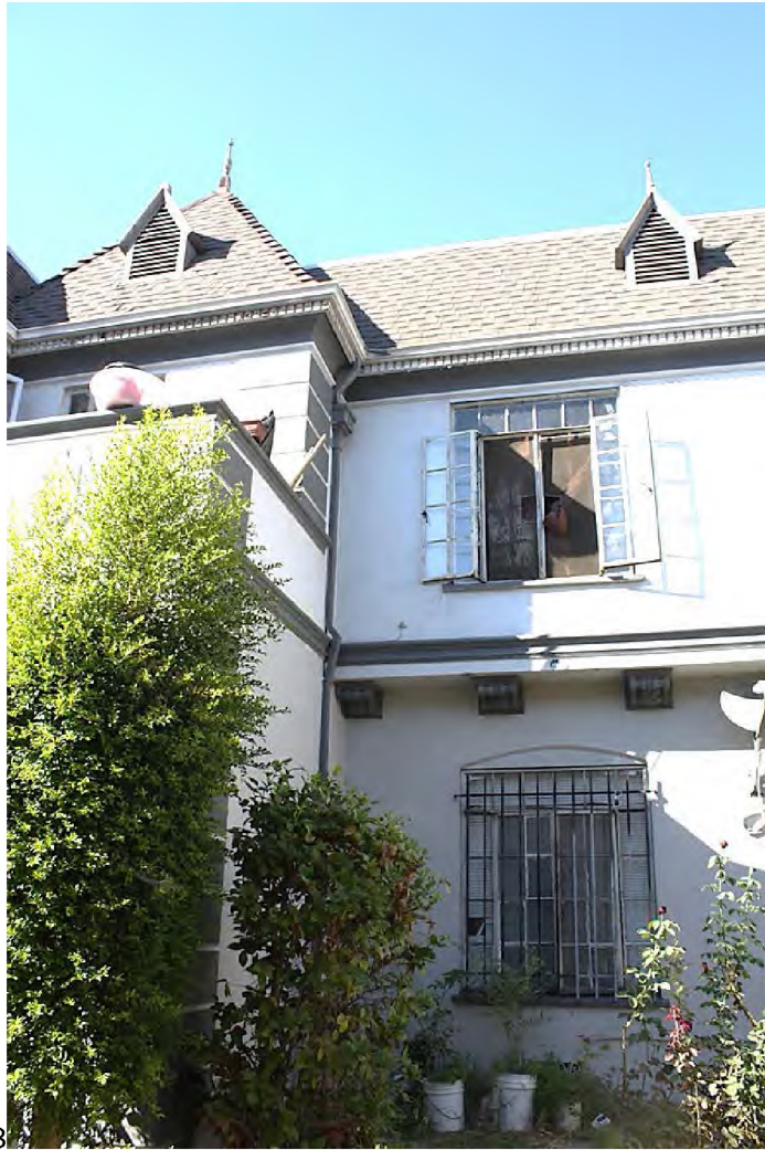
Balcony, south façade steeply pitched roof with gabled vents, pinnacles; steel frame casement windows, fixed transoms; view north.
