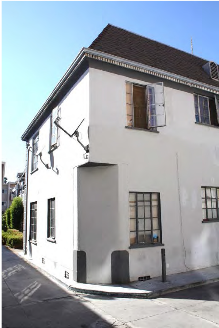
South elevation of rear portion with corner cut at southeast corner, corner buffers & curbing to protect building; partial east elevation; steel frame casements, view northwest.
