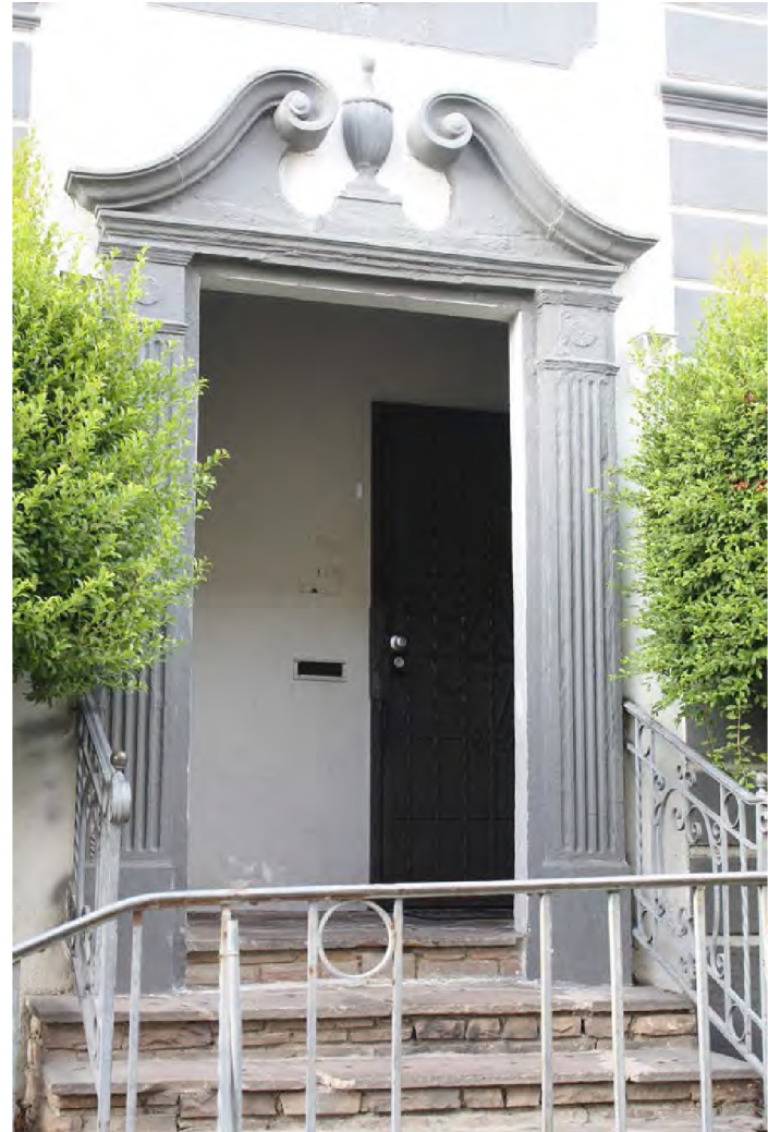
Raised entrance to west/front units: Balustrade of entry steps; French stone steps with decorative balustrades; entry surround with piers, broken pediment with urn; cast decorative panel; banding; quoining; view north.
