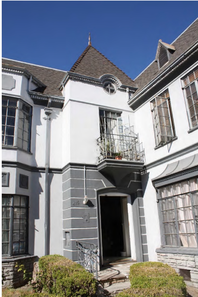
Raised entrance to unit 416: Extended quoining forms entry, goes around cantilevered balcony with wrought iron patterned balustrade, banding, dentil, pinnaced gable with inset oculus, view northeast.
