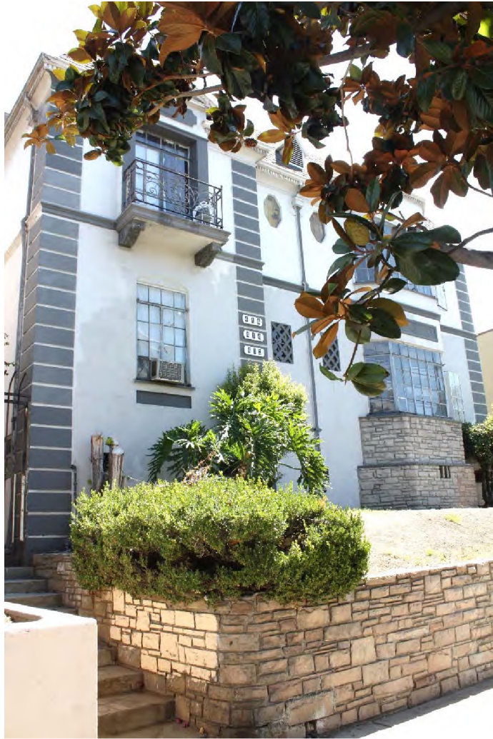
Building west elevation: French stone retaining wall; quoining; cast decorative panel; balconette w/ wrought iron balustrade, brackets, banding; steel frame casement windows; octagonal window; diamond window grille; French stone bay window base, view southeast.
