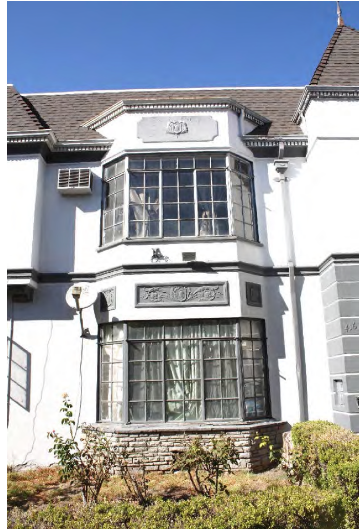
First bay of steel frame casement windows to the south of Catalina on south elevation: French stone base, stucco decorative panels, banding, dentil trim at hipped roof with flat deck, gutter/downspouts, view north.
