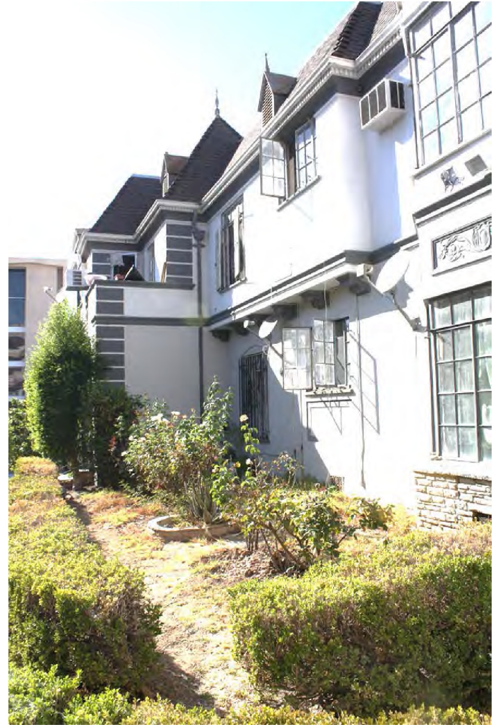
View along south façade of building: Balcony of upper west unit; quoining; steeply pitched roof; pinnaced gables; casement windows; French stone trim, window bay; banding; dentils; cantilevered 2 nd story & brackets; cast trim panels; view west.
