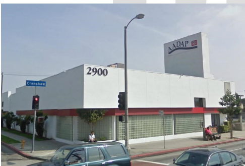
Example of architectural feature originally designed to accept signage.
