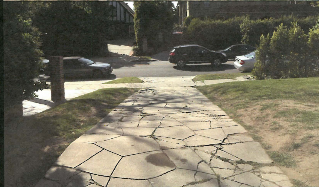
Slope too steep for ADA wheelchair access compliance and leads straight onto busy thoroughfare of Rossmore Ave
