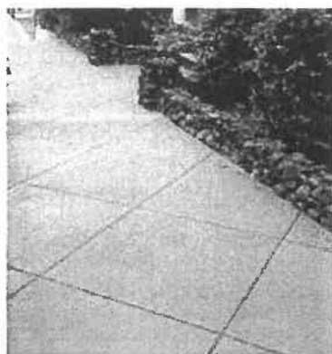
Figure AA.2 Cast-in-place scored concrete
