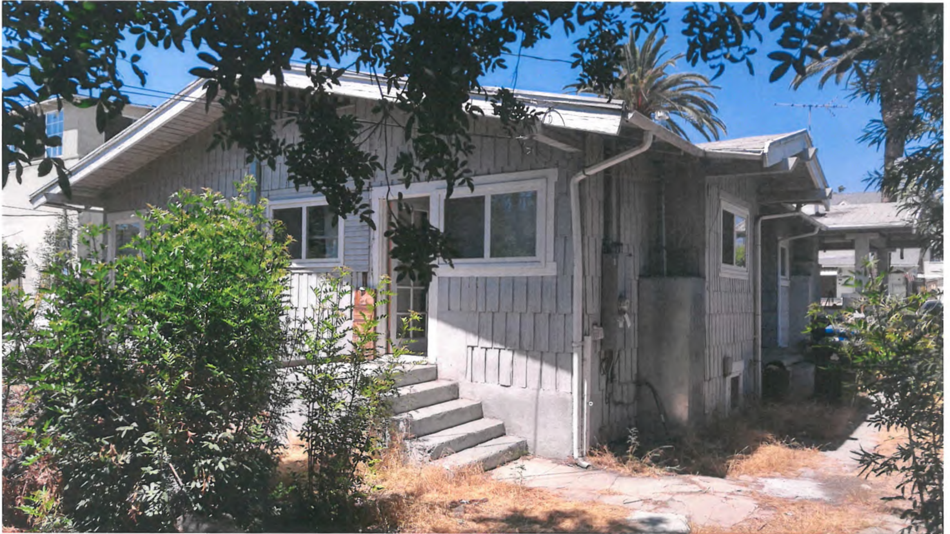
Rear and side façades of 4406 West Kingswell Avenue, August 11, 2016.
