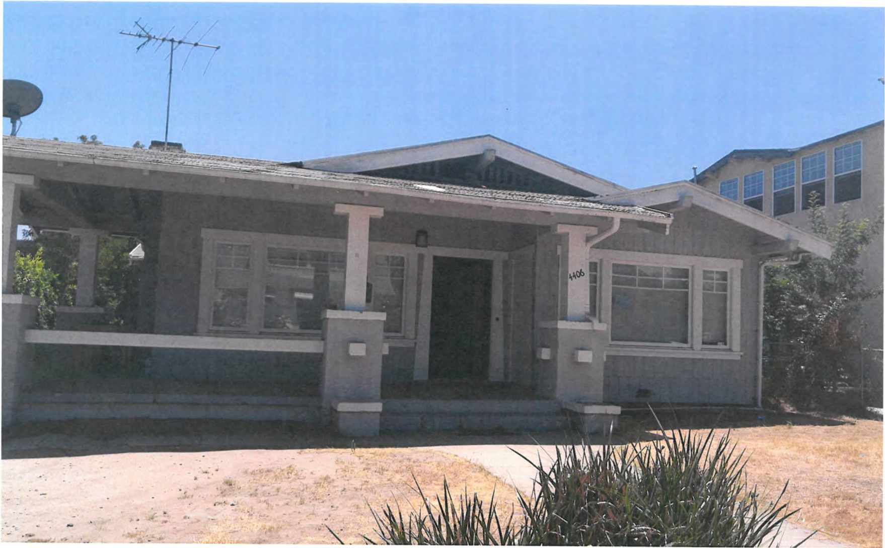
Front façade of 4406 West Kingswell Avenue, August 11, 2016.
