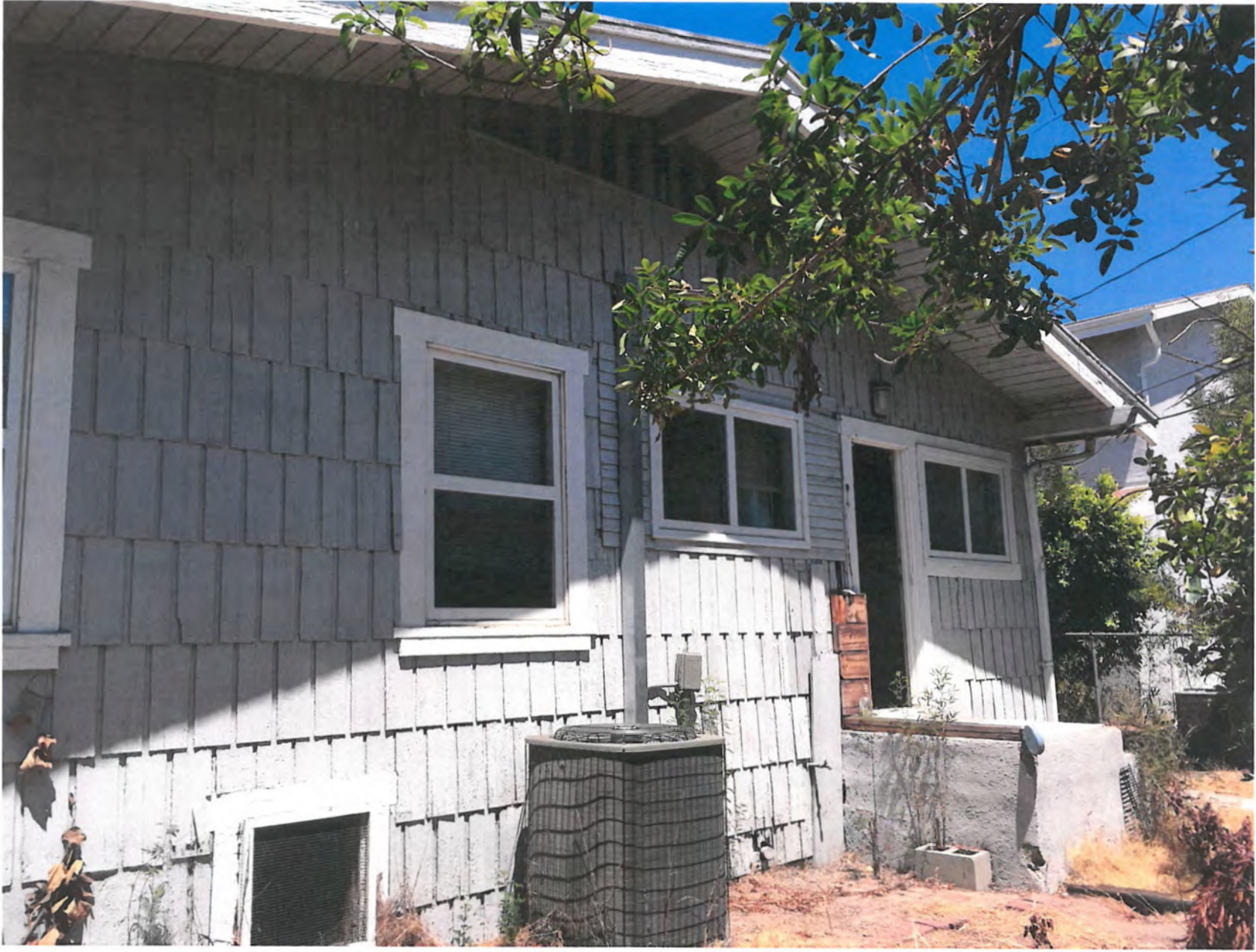
Rear façades of 4406 West Kingswell Avenue, August 11, 2016.
