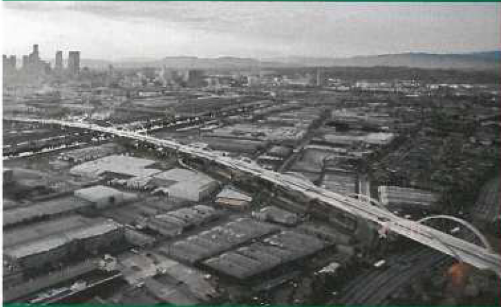
Sixth St Viaduct Replacement
