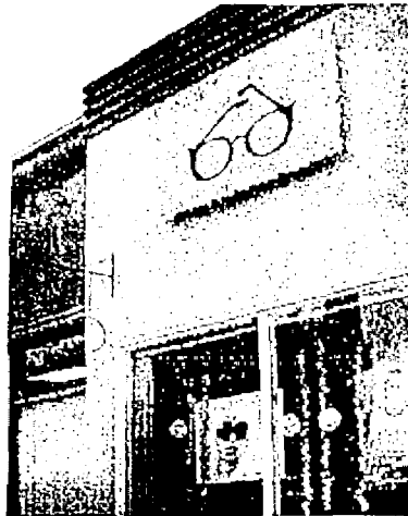
Logo laser cut out of metal panel, held off from building and halo lit creative use of design and material for distinctive business identification.
