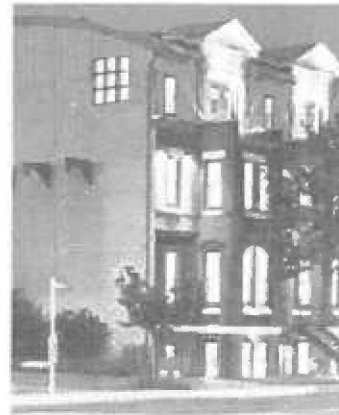
As described under leaves in Washington D.C., a substantial amount of the original materials could not be salvaged. Therefore new, more industrial materials were introduced where historic fabric was missing, and a addition was designed for the rear end roof of the original historic building.
