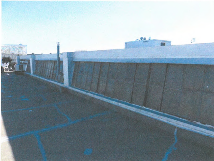
Monitor roofs have original steel sash.
