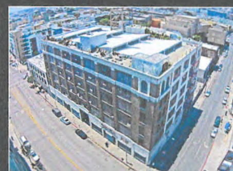
Catalina Swimwear Building Now: Fifth & San Pedro (Built 1923 - 443 S San Pedro St)
