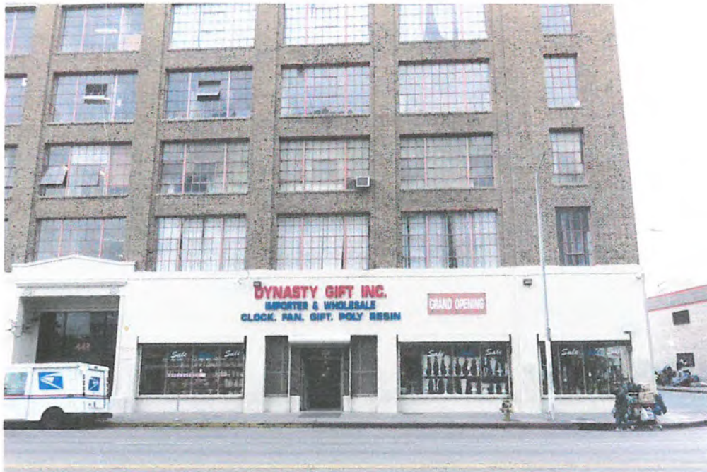
Former storefront openings conform to window placement on upper façade. Original pediment remains over recessed central entrance.
