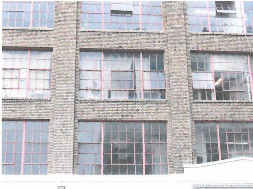
Steel sash on upper façade are original, and in fair condition. Note awning operation of center sash
