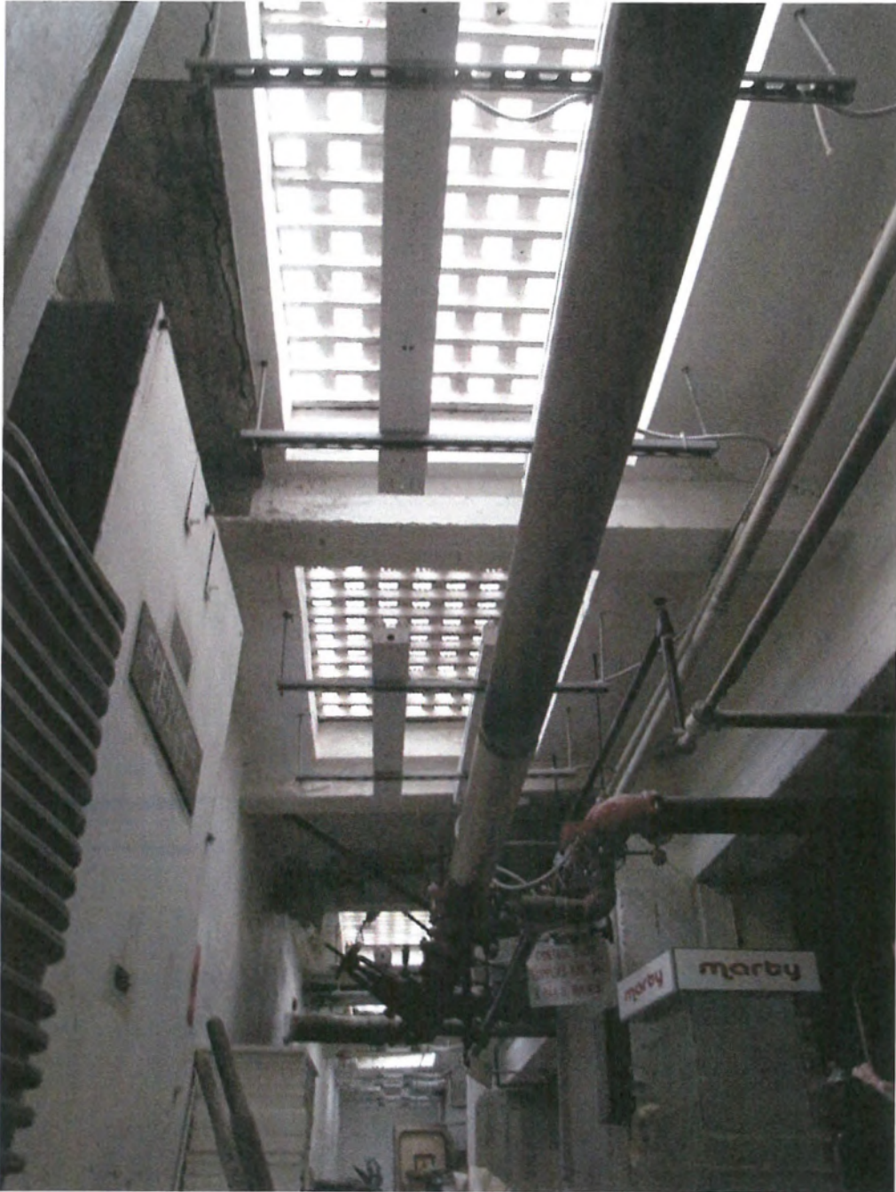
Figure 22. View looking up at the vault lights along the western wall of the basement level.
