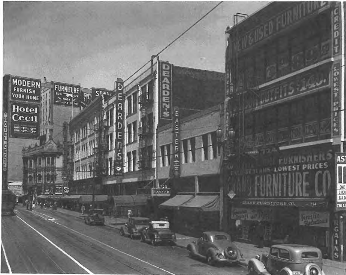
Figure 11 Looking at south elevation of Hotel Cecil, showing historic usage of painted wall signage for off-site advertising, and the original blade sign also appears to the left edge of photo.
