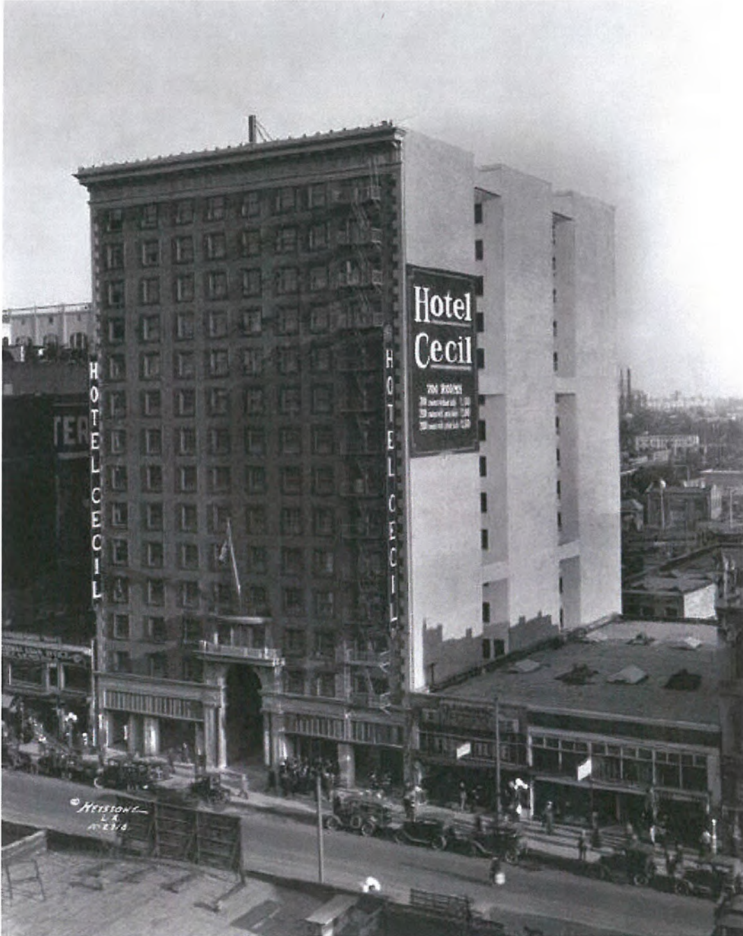
Figure 9: Undated black and white photograph showing the west (S Main St) and south elevations of Hotel Cecil.
