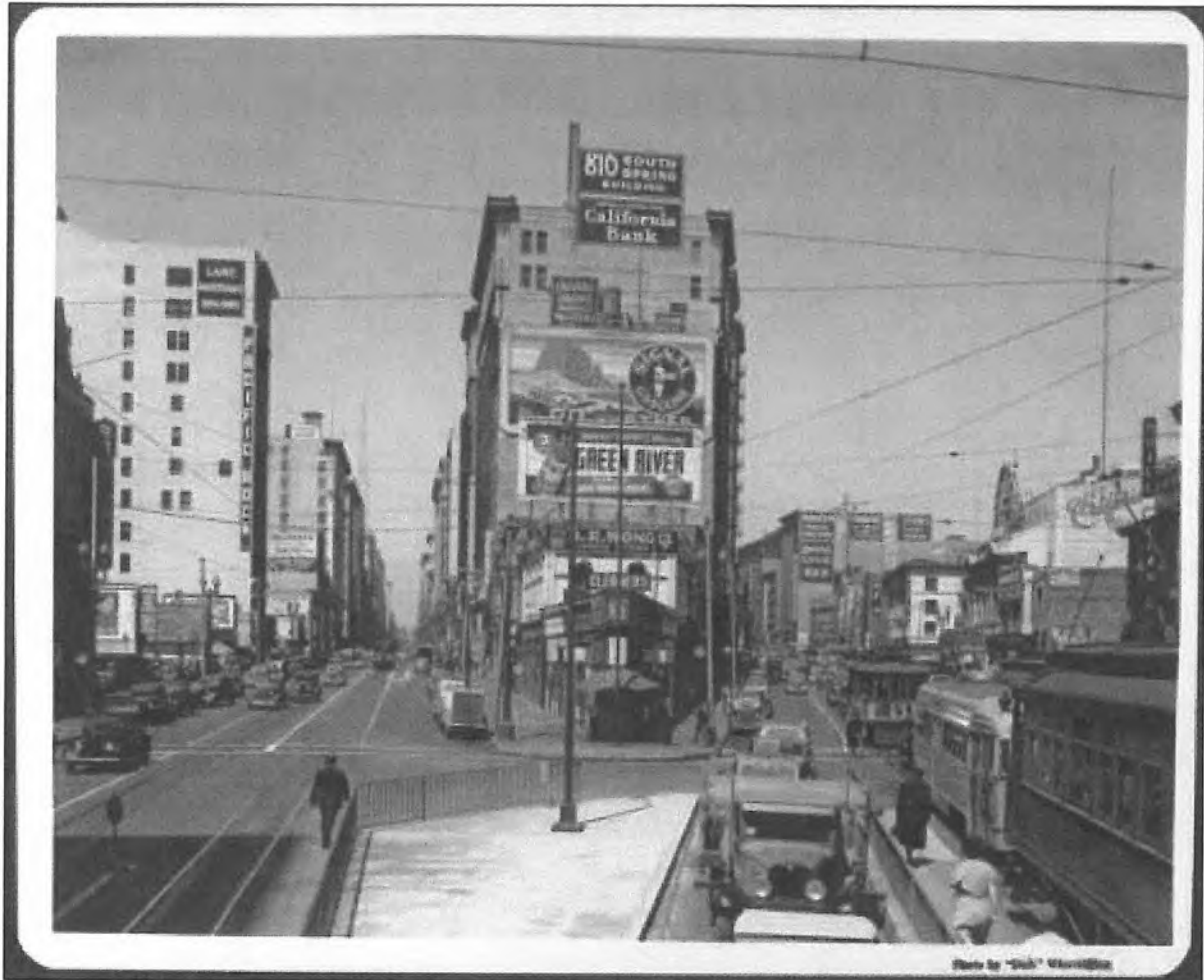
Figure 10: South elevation of Hotel Cecil appears in the right rear of image. Note the use of painted wall signage used for off-site advertising.'
