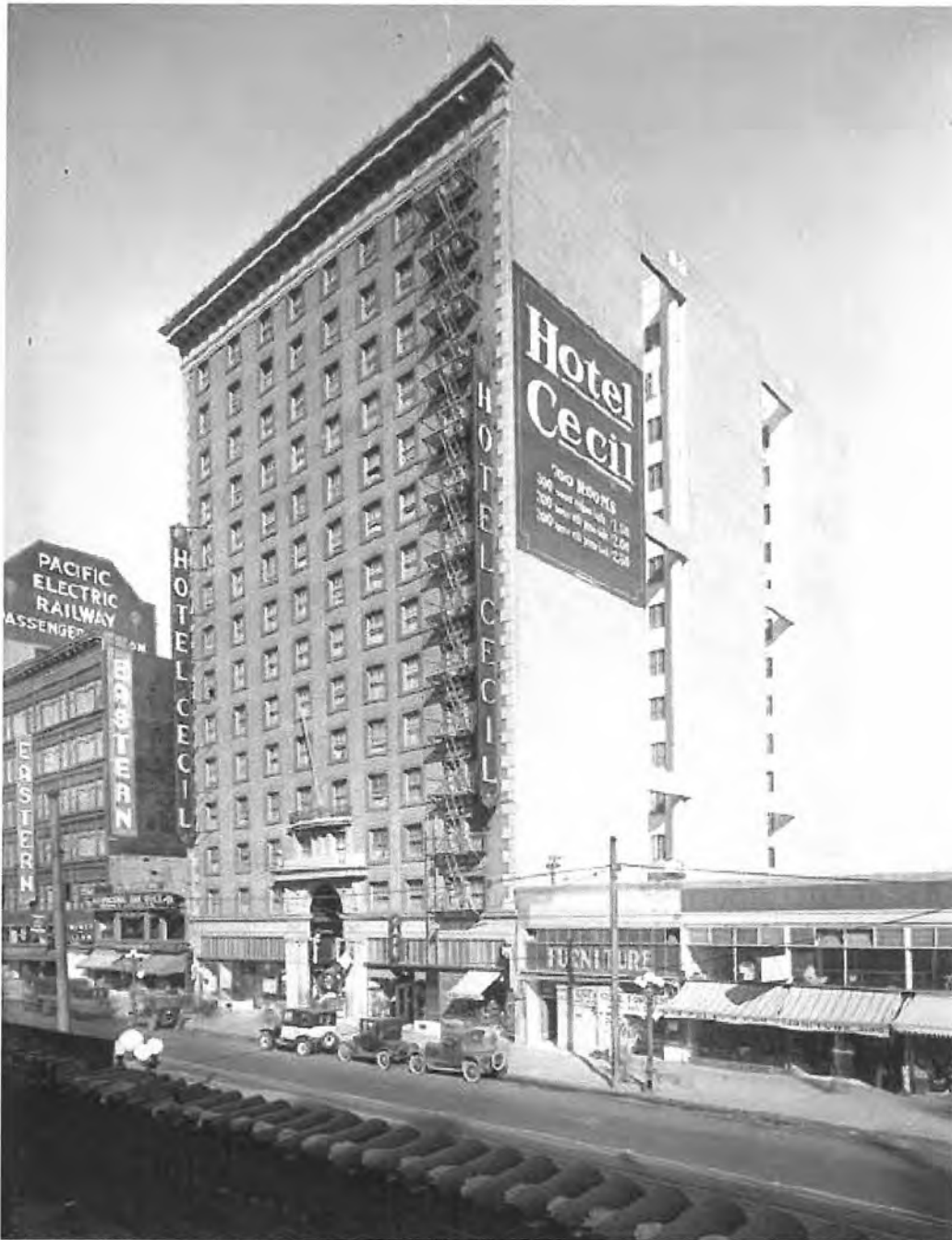
Figure 8: Undated black and white photograph showing the front (S Main St) and south elevations of Hotel Cecil. The advertisement painted on the south elevation of the building indicates Hotel Cecil as having 700 rooms, a fact that is discredited by early occupancy permits and the historic architectural drawings.
