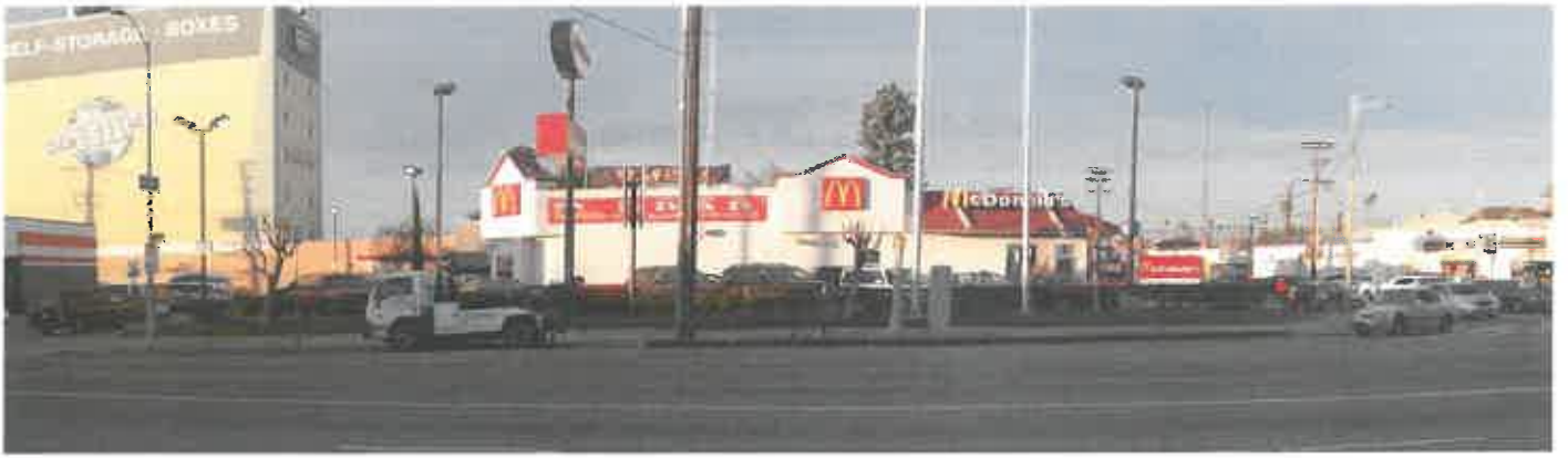
19. McDonald's restaurant abutting across Washington Boulevard to the north.
