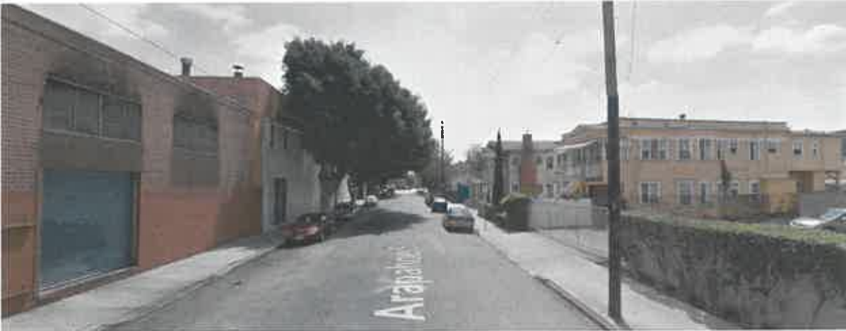
6. Multiple family residential along the southerly portion of Arapahoe across from proposed parking and landscaped buffer.
