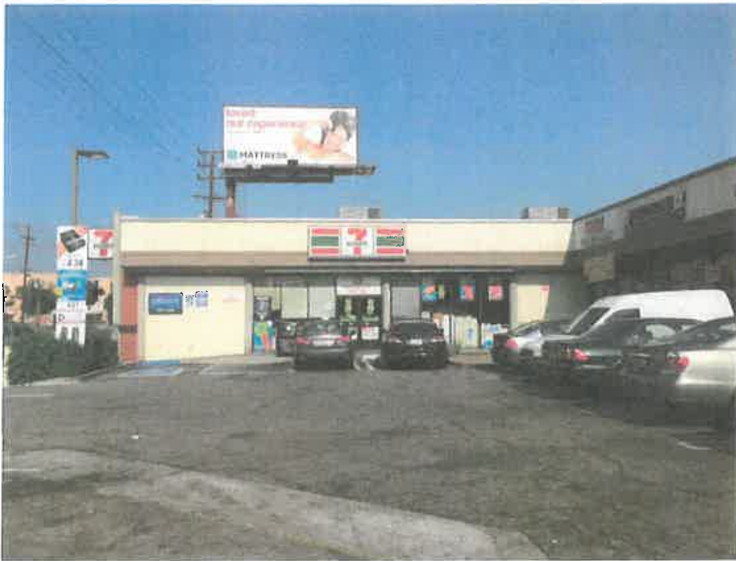
1. 12450A Burbank Blvd: view looking east at the front entrance of the subject site.
