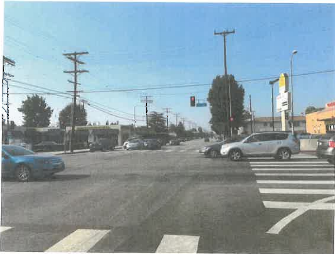
15. 12450A Burbank Blvd: looking north onto Whitsett Avenue.
