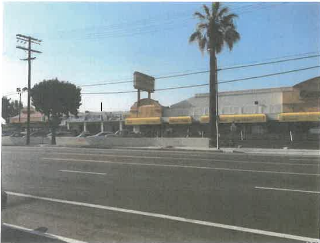
17. 12450A Burbank Blvd: view looking north at the neighboring businesses to the north of the property.
