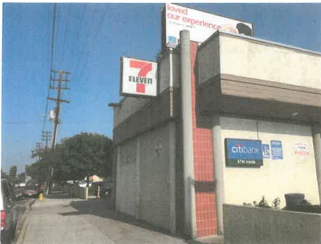
3. 12450A Burbank Blvd: View looking southeast at the north side of the subject property.
