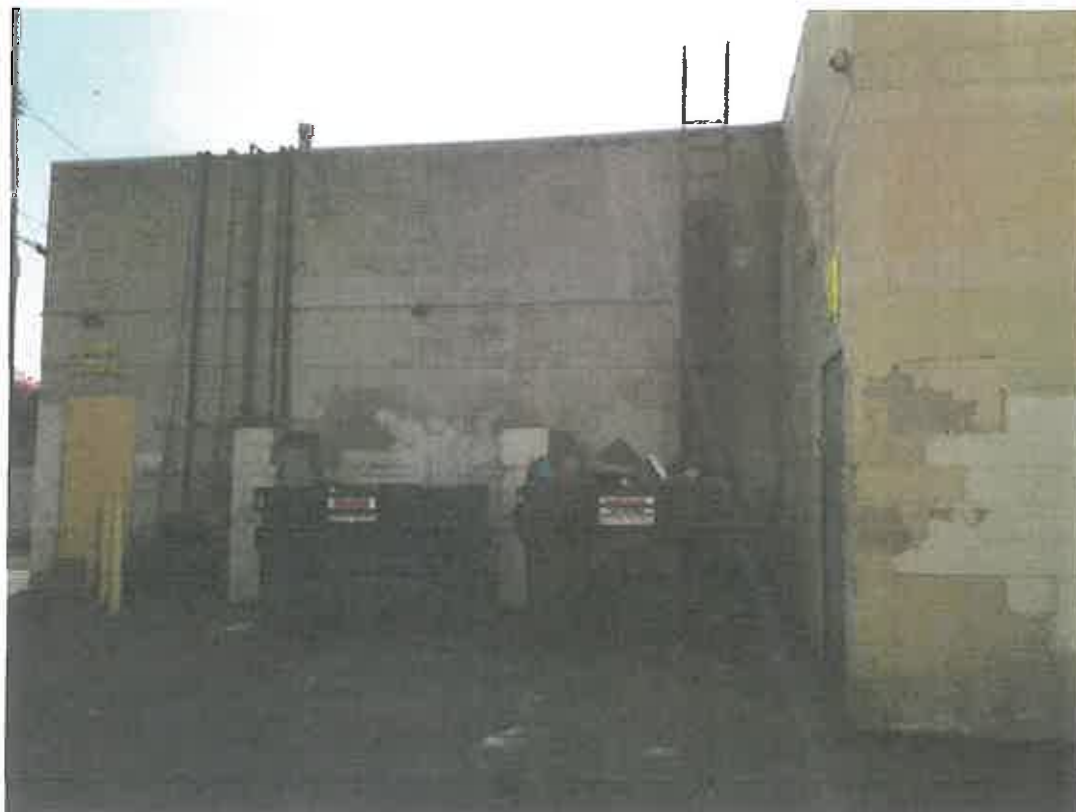
6. 12450A Burbank Blvd: view looking west at the trash bins on the east side of the property.
