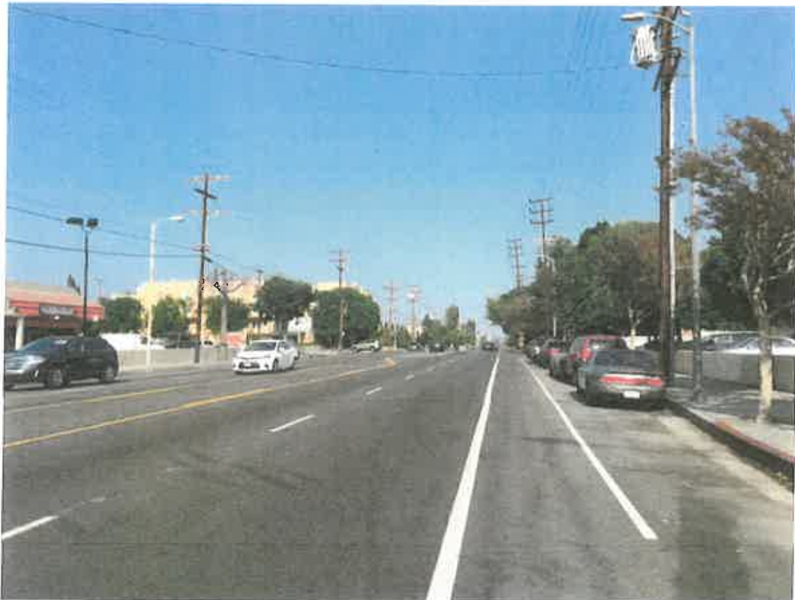
12. 12450A Burbank Blvd: looking east onto Burbank Blvd.
