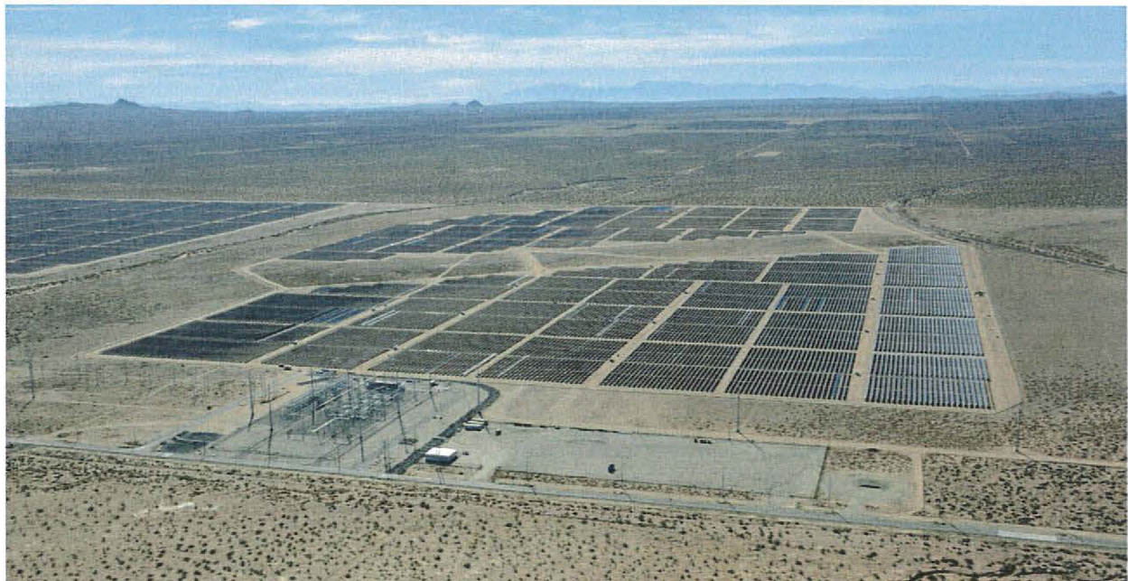
Beacon Solar Collector Station and Site 4 (January 31, 2017)
