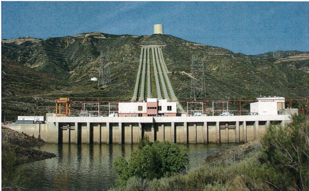
Front view of Castaic Pumped Storage Plant
