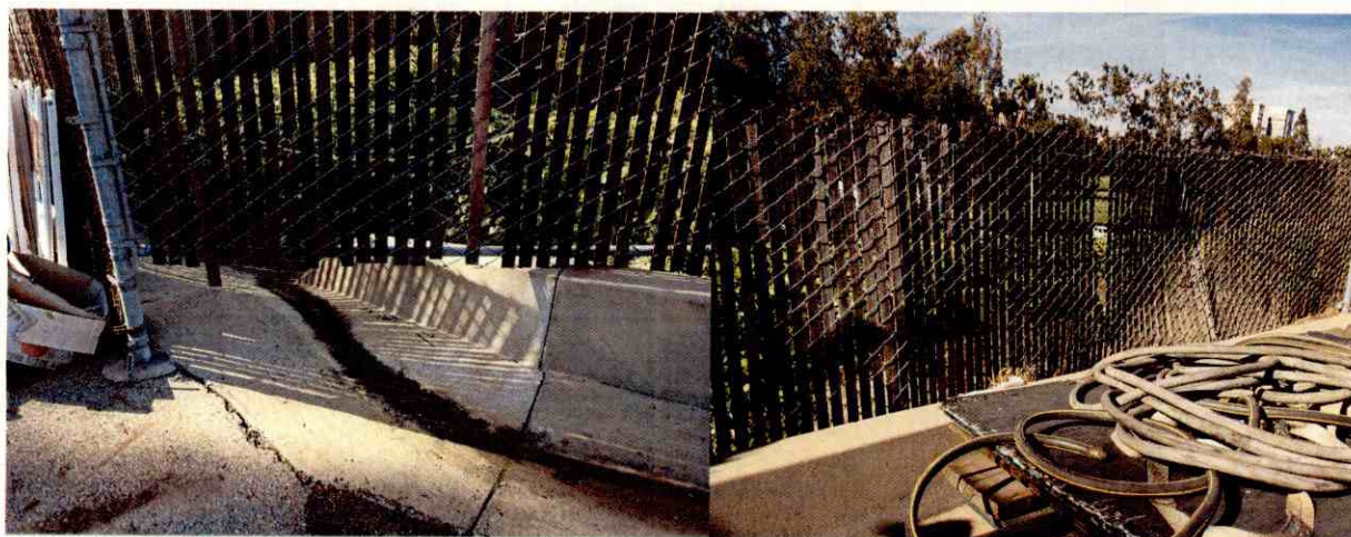
Figure 3. Displays "Fencing Violation Area #2". The drainage system is not fenced or covered and may create access into the facility. In addition, several sections of fencing in this area is damaged.
