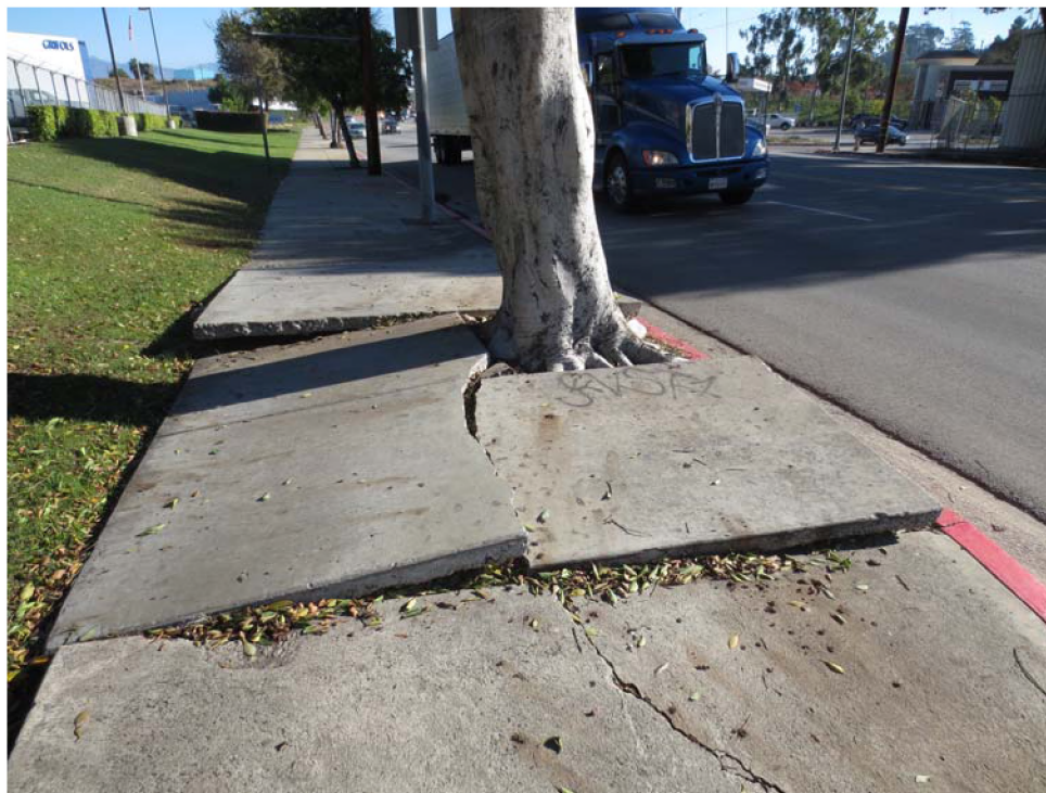
FIGURE 7 – SIDEWALK LIFTING, VALLEY BOULEVARD
