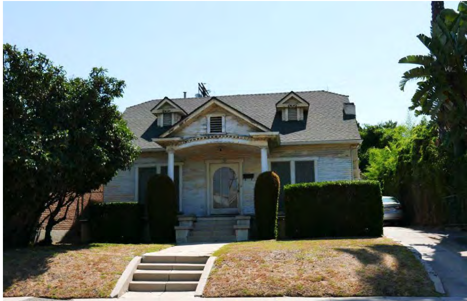
Figure 11. Frontal View of 646 N. Gower Street Property SOURCE: Sapphos Environmental, Inc., 2017
