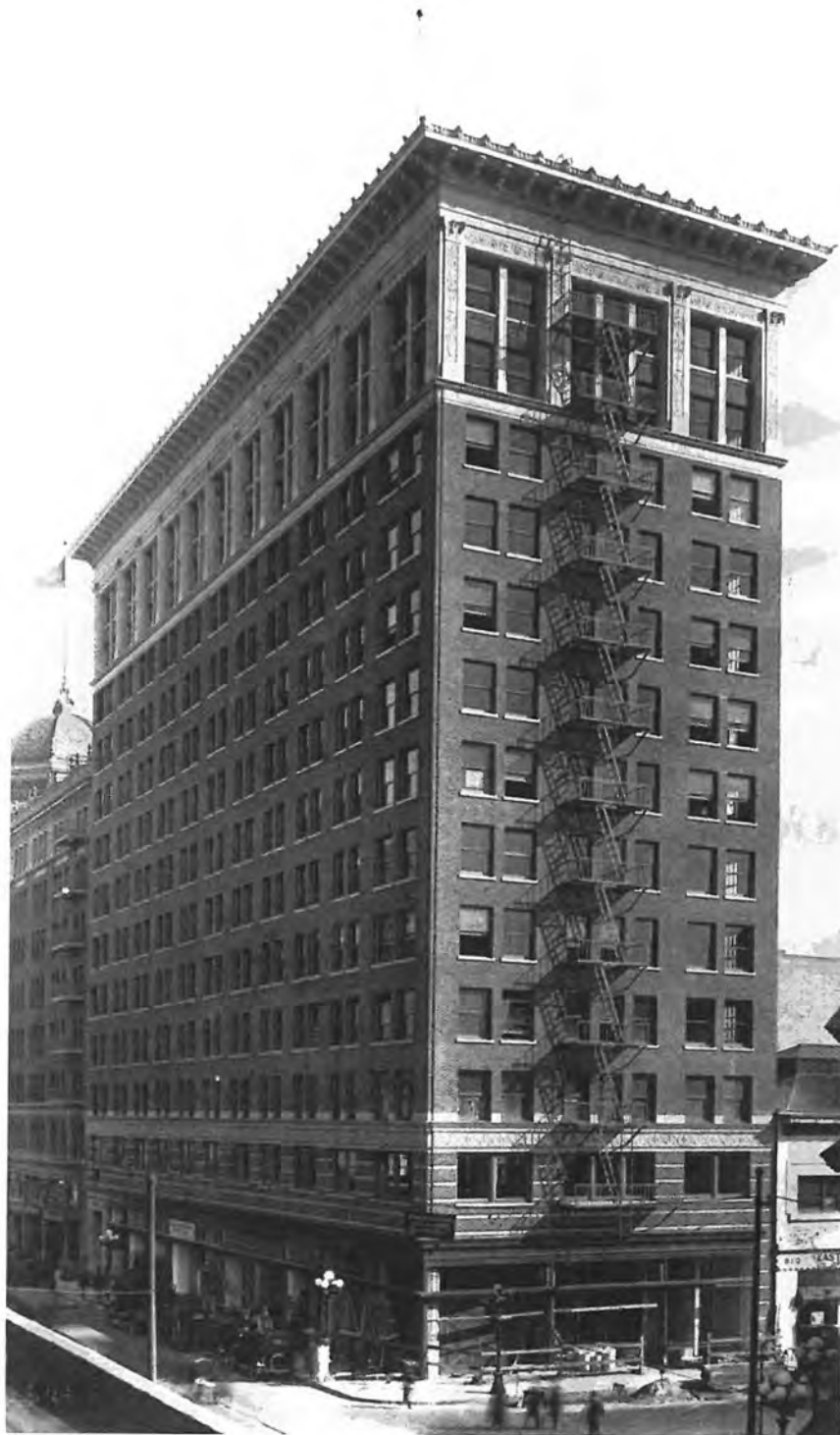
Image 1 Commercial Exchange Building, nearing completion in 1924, showing final assembly of original storefront design and configuration. This image is the basis for the 2016 rehabilitation.
