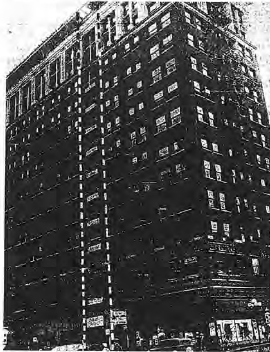
The thirteen-story, height-limit Commercial Exchange Building at Eighth and Olive streets is being sliced in half to conform to the setback line of Olive street. Superimposed dotted lines indicate the ten-foot section which is being removed.
