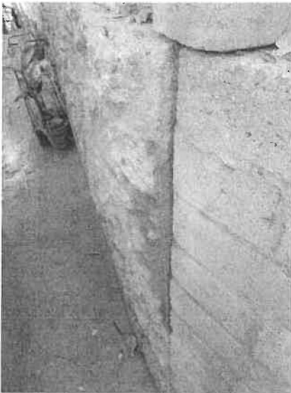
Indication of earth movement below grade.
