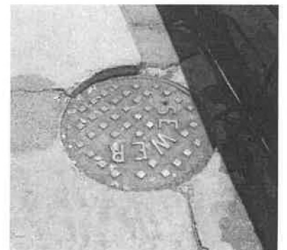
Above right: Concrete above curb on Edgemont St. shows earth movement
