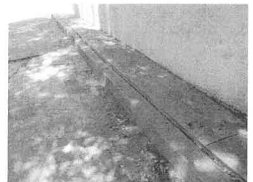
Above right: Concrete above curb on Edgemont St. shows earth movement
