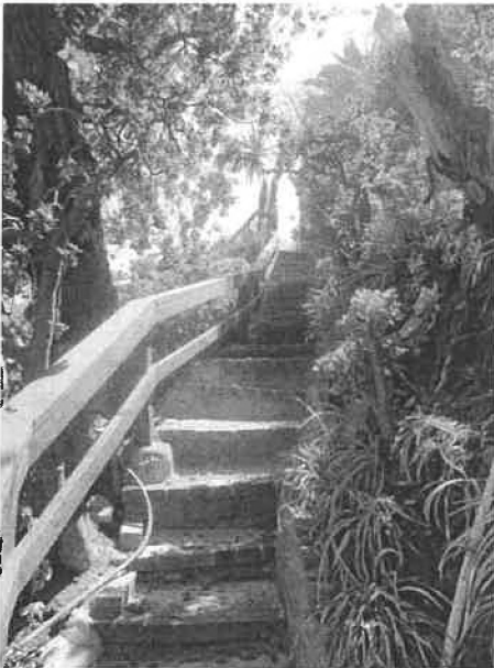
Excavated stairs along hillside that were completely buried by previous slide.
