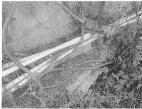
Footings of retaining wall at property line exposed due to earth movement.
