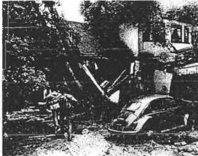
PRECARIOUS —House at 3843 Tujunga Terrace in Hollywood looms against tree after landslide at backyard pushed it off foundation. Tree is keeping house from sliding down into another. Photo taken by Cal Newsphoto.
