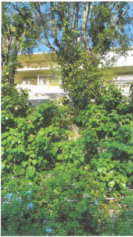
Above: Photo taken from bedroom window showing retaining wall, terraces and 2937 Glendower property excavation site.
