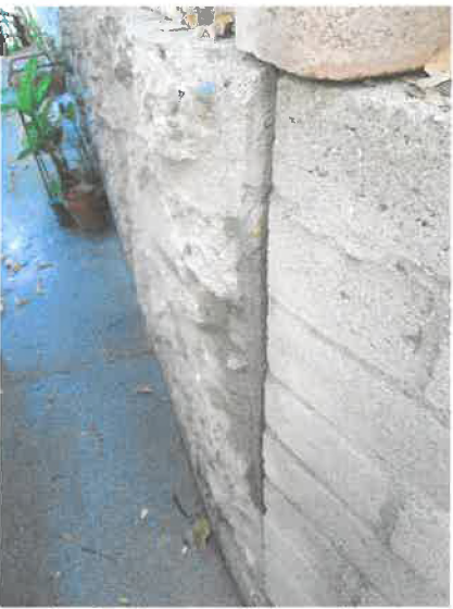
Indication of earth movement below grade.
