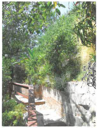
Photo shows hillside prone to landslides.
