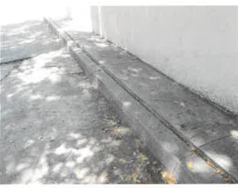
Above right: Concrete above curb on Edgemont St. shows earth movement
