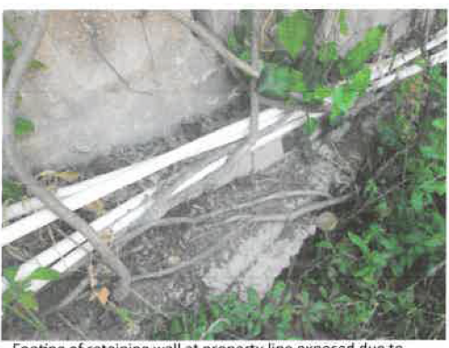
Footing of retaining wall at property line exposed due to earth movement.
